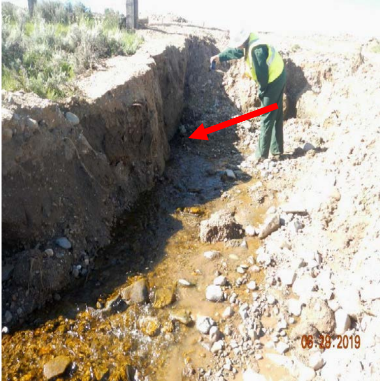
Photo#12: Close view of NE washout. Arrow indicates point where water is discharging in Photo#13.
