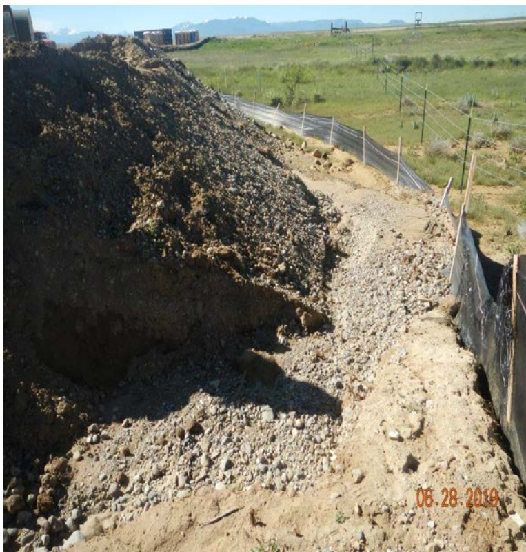
Photo#5: View of NW washout from bottom of slope and overwhelmed silt fence.
