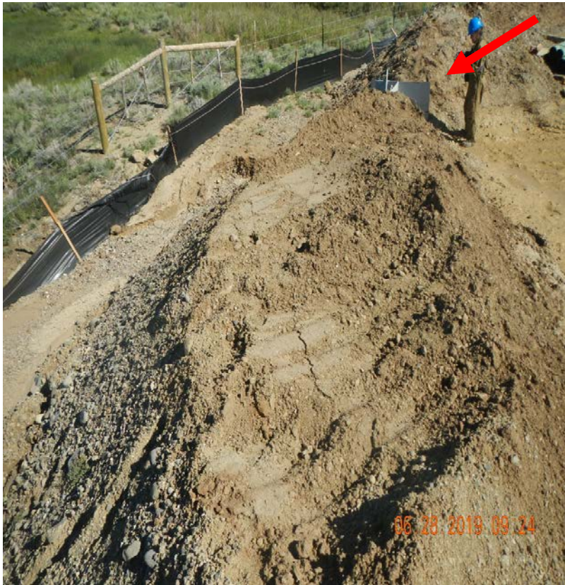
Photo#3: Area where washout occurred at Northwest corner. Arrow indicating Weir in Photo#4
