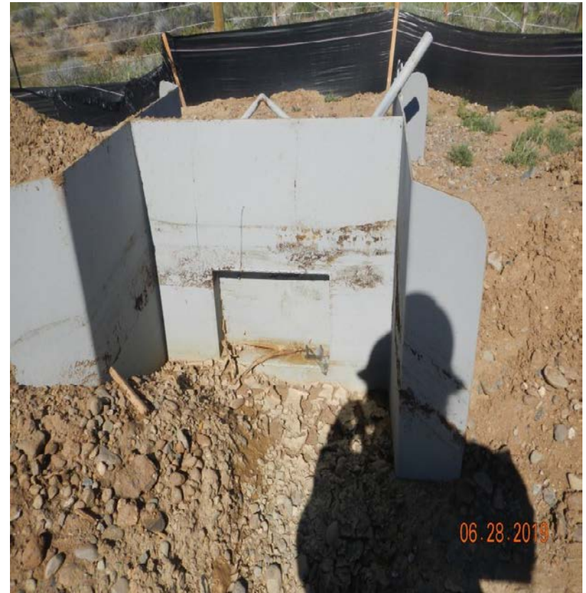
Photo#4: Weir installation, at area where washout occurred at Northwest corner.
