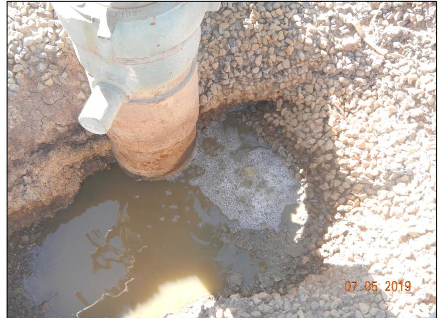
Photo #4 Photo at Wellhead. Bubbles coming from around wellhead inside of cellar
