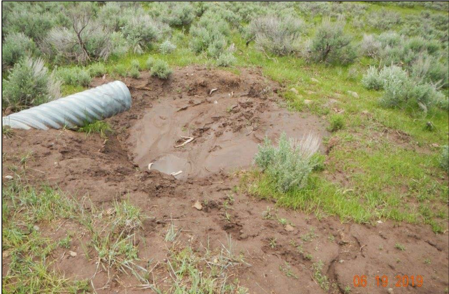
Photo 3. View of silt trap at culvert outlet along access road. Silt trap is full of sediment, overflow outlet not observable, rilling from roadside evident. Culvert installed above grade will accelerate erosion and needs outlet protection.
