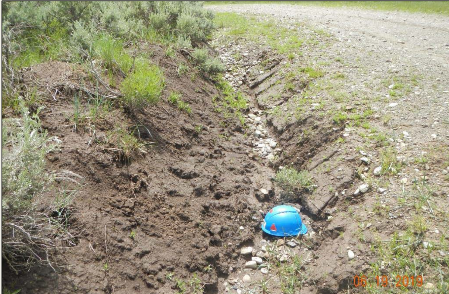
Photo 2. View of erosional channeling and rilling along the access road near the well pad entrance. Ditch banks are not stabilized.
