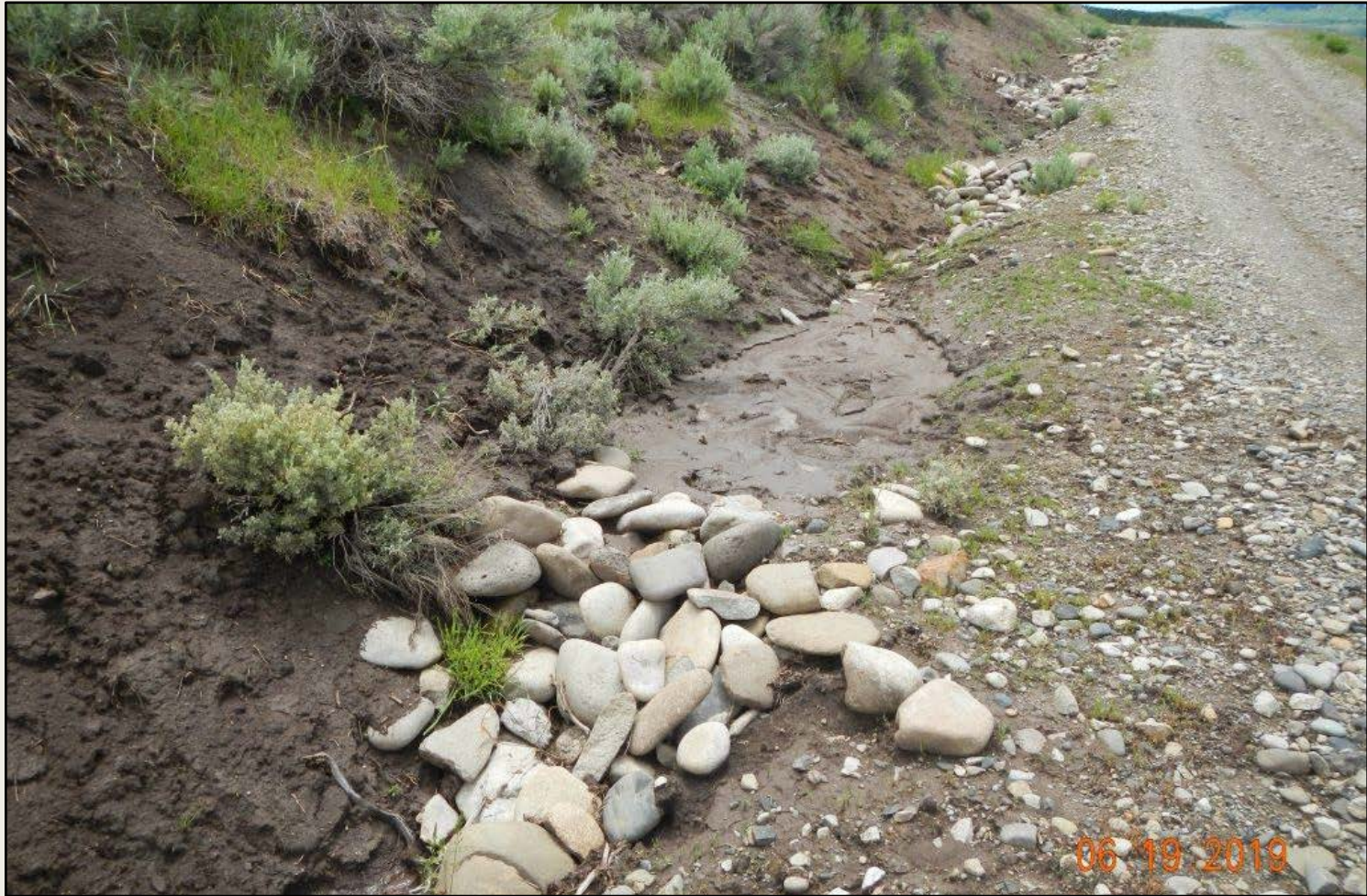
Photo 6. View of cobble check dams along the access road, not installed using good engineering practices. Sediment is accumulating above the rock and erosional channeling is occurring downstream.
