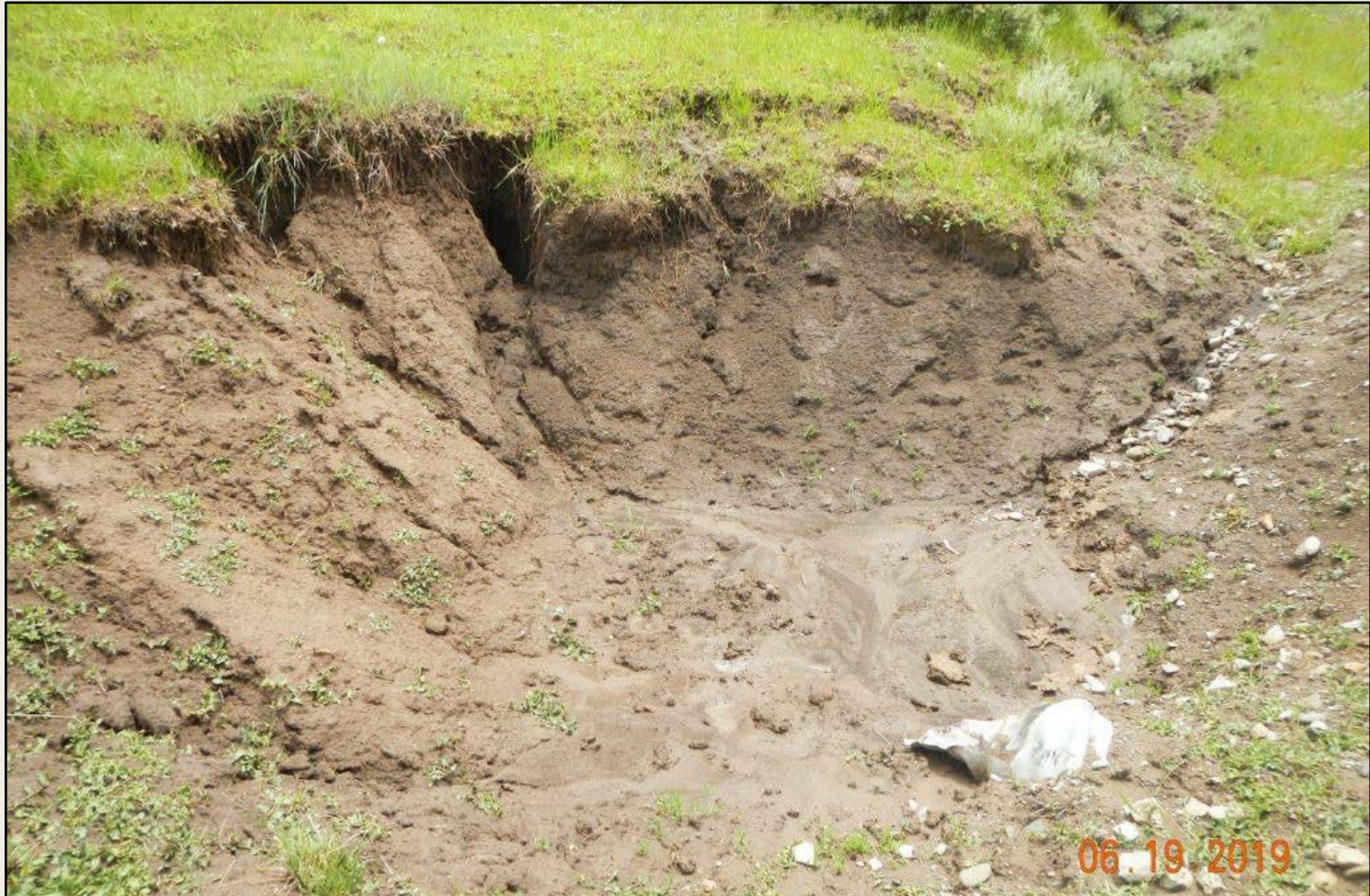
Photo 5. View of bare, eroding soils at culvert inlet, erosional channeling and sedimentation at silt trap at culvert inlet along the access road. Culvert is full of sediment.
