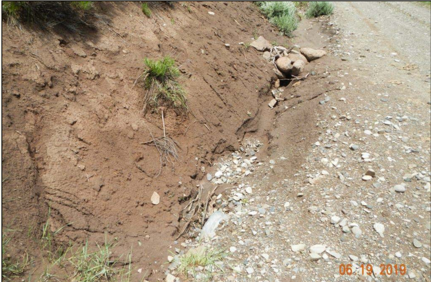
Photo 4. View of erosional channeling, rock check that is inadequate and not properly installed, along the access road. Bare soil on cut-slope are not stable.
