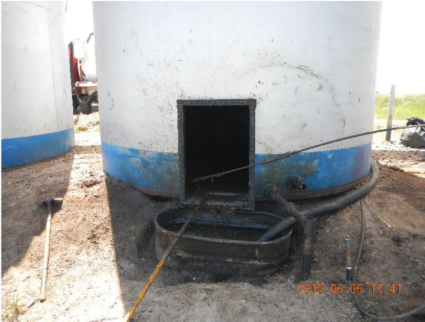
Photo 3: Hatch and flame tube removed from tank.
