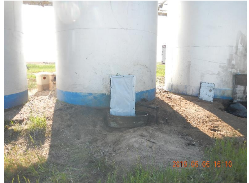
Photo 4: Plastic sheeting installed over entry hatch.
