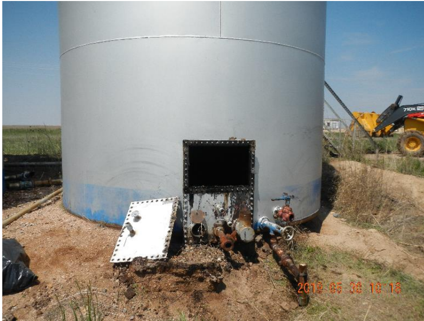
Photo 15: Entry hatch removed from P3.
