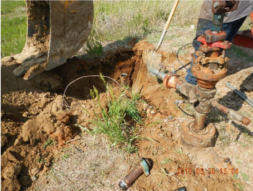
Photo 19: Disconnecting flow line from wellhead.
