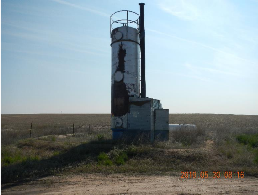
Photo 9: Vertical separator and shed.
