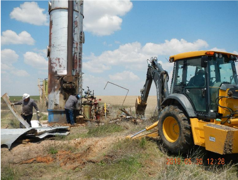
Photo 17: Tearing down separator shed.
