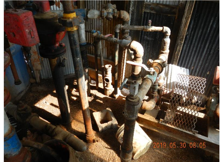
Photo 8: Flow lines and transfer pump inside separator shed.
