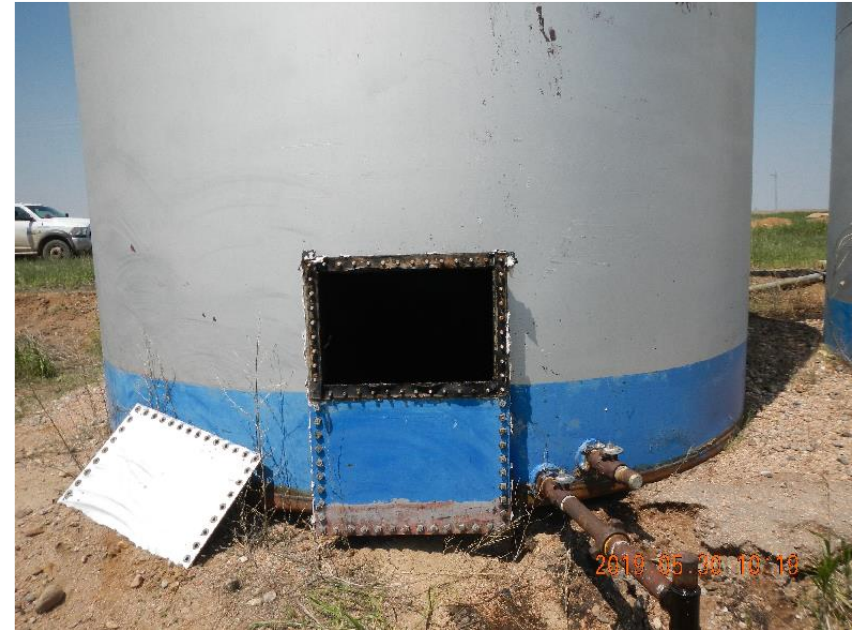
Photo 16: Entry hatch removed from P1.
