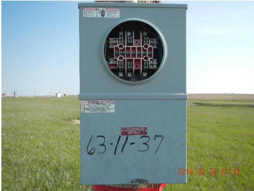
Photo 3: Power supply box with removed power meter.
