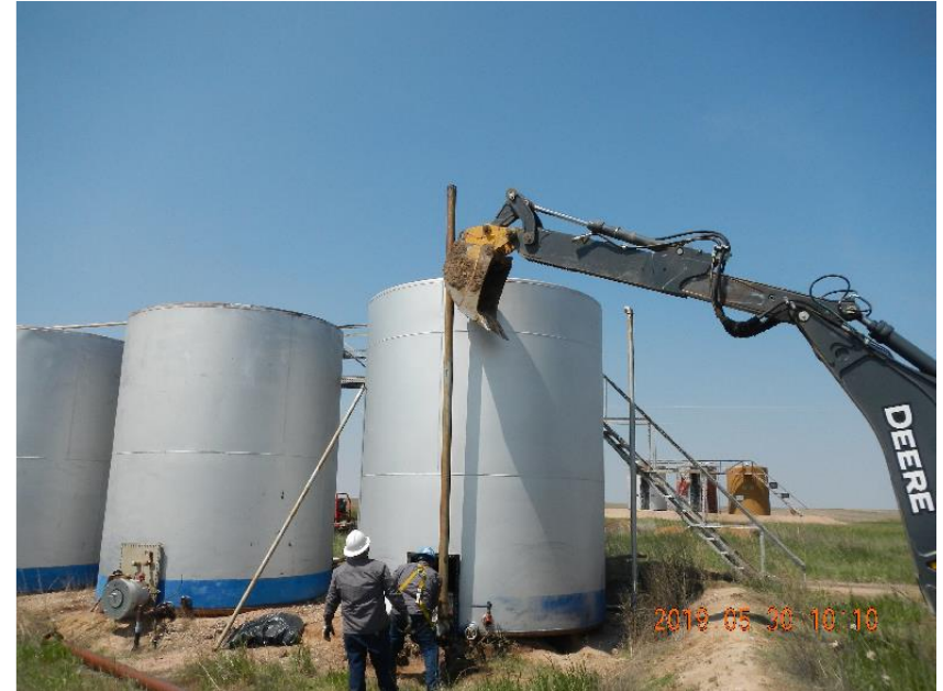
Photo 4: Removing the heater vent stacks off the oil production tanks.
