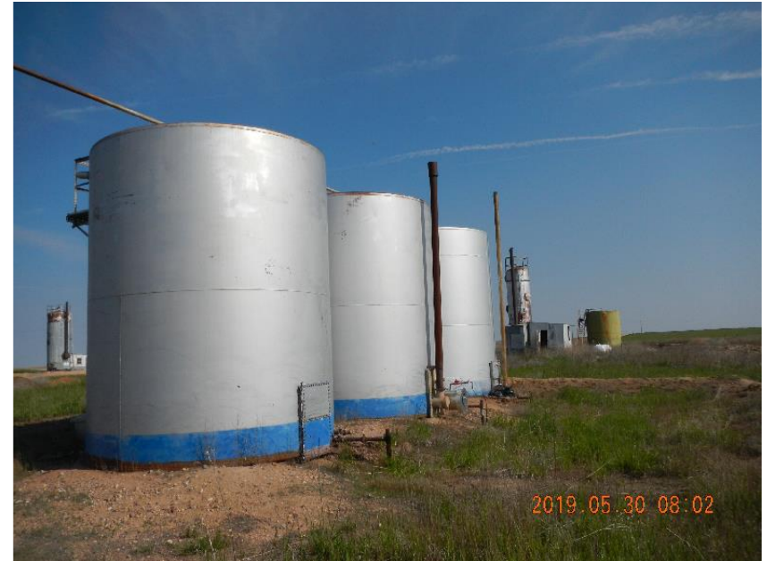
Photo 6: Oil production tanks with water tank in background.
