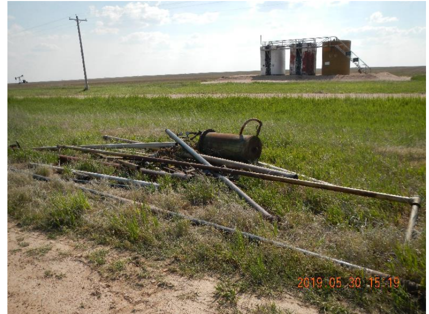
Photo 22: Tank piping piled and ready for loading and haul off.
