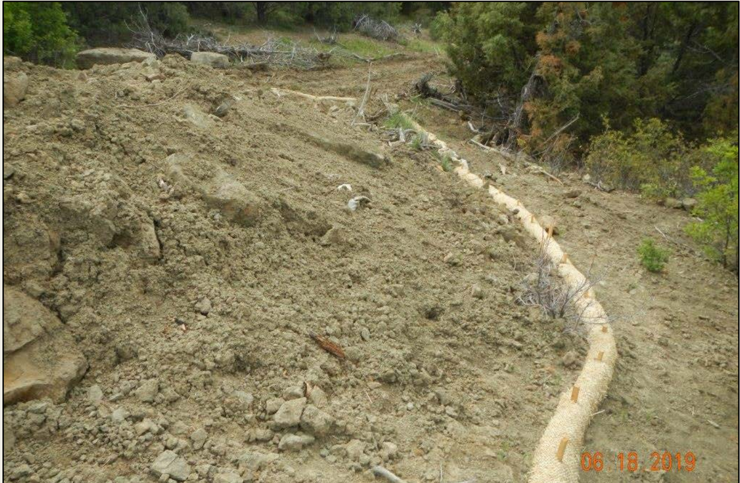
Photo 2. View of wattle at spill site. This wattle is not sufficient to contain volume of excavated soil above slope. Disturbed soils down-slope are not stabilized.
