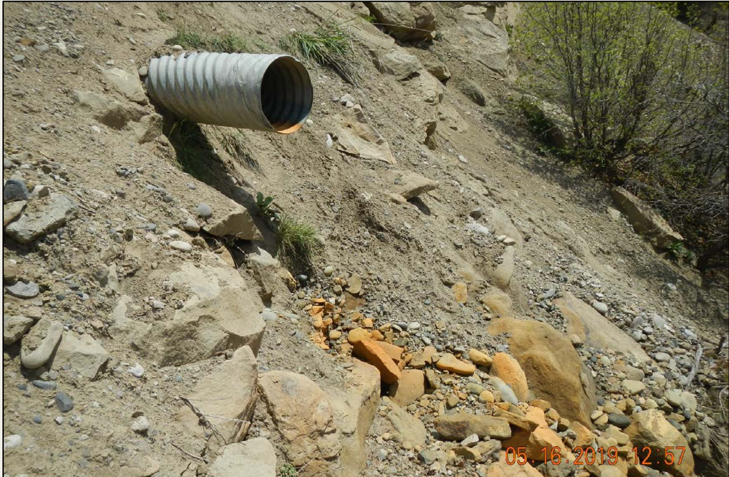
Photo 12. View of culvert outlet down-slope from release that shows discolored rock and soil indicating impacted material is flowing off and down from the release area.
