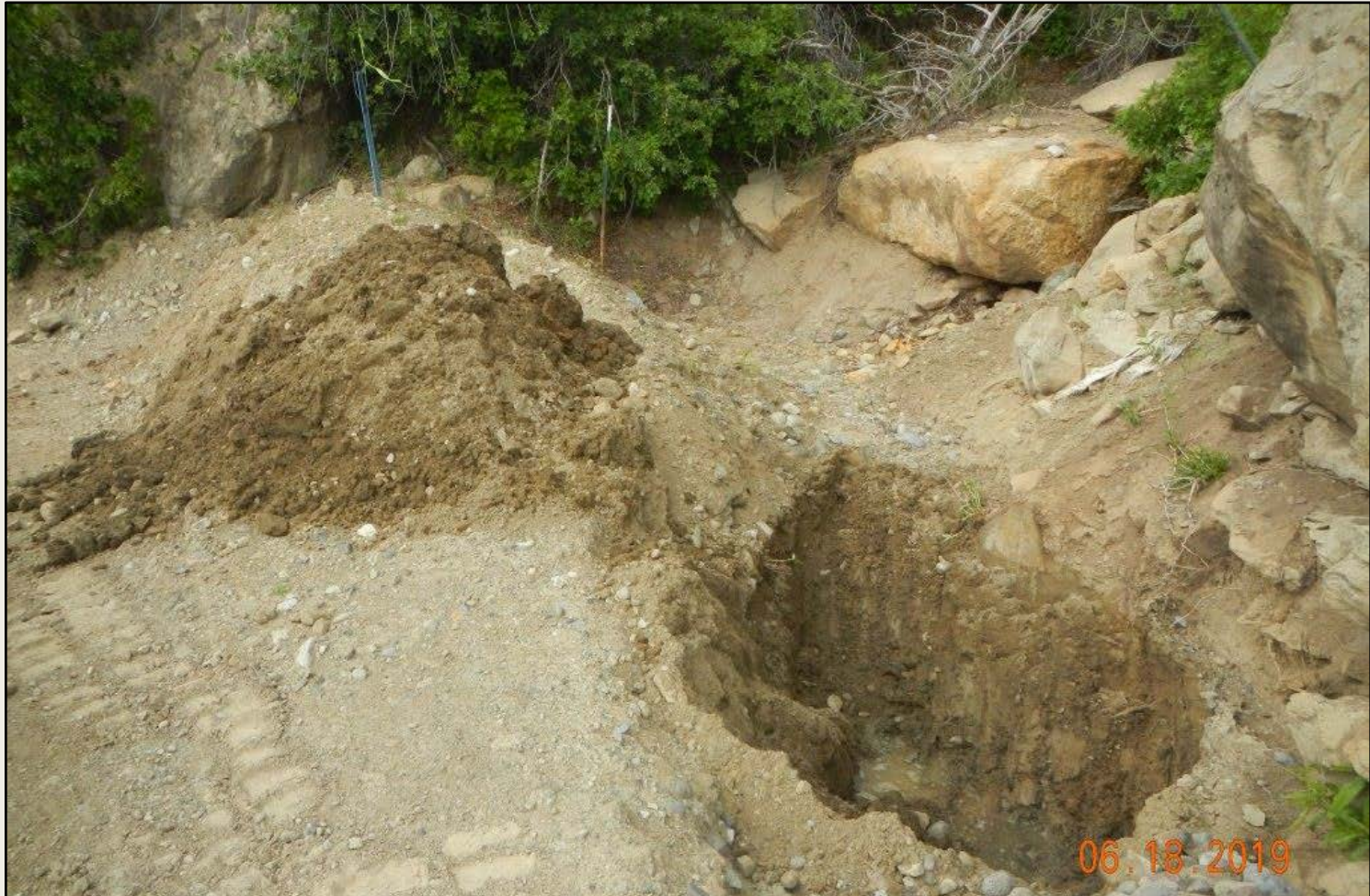
Photo 1. View of loose excavated soil and trench downstream from spill along access road. Stormwater controls are needed around stockpiled soils to prevent sediment transport.
