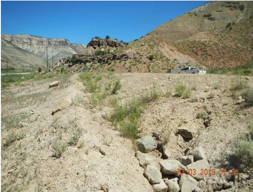
Washing and movement of sediment in ditch at front of location.
