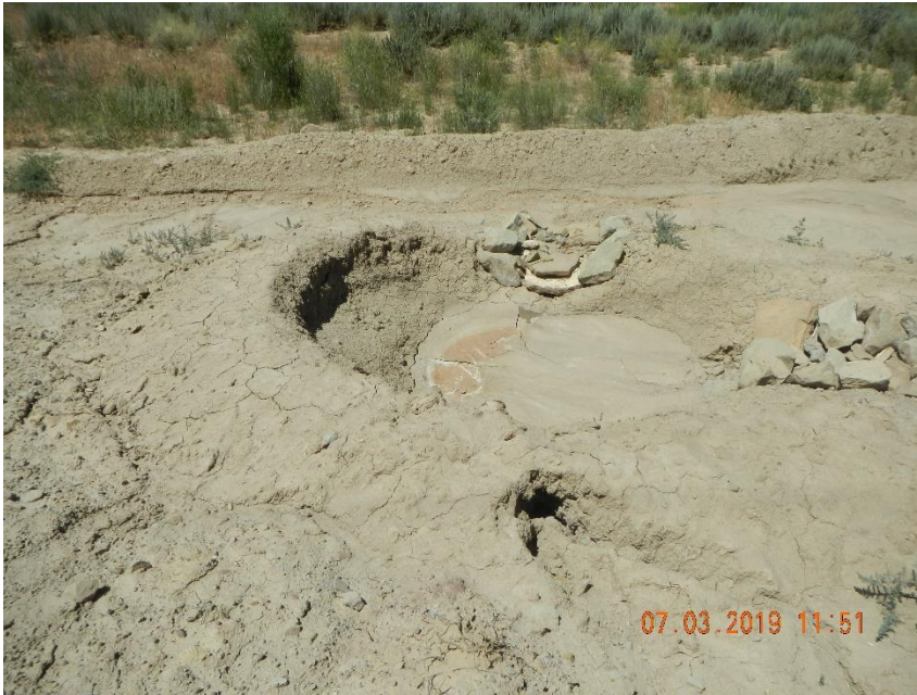
Channeling of check dam wall.
