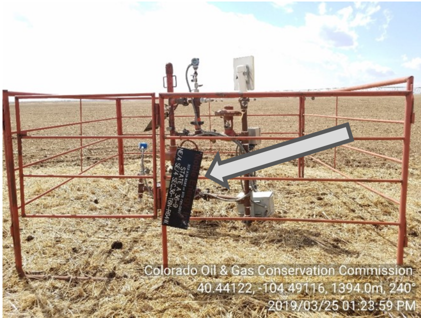
Photo #1 State A 36-9 (05-123-14790) Wellsite Shut-In | SI Emergency Contact number NOT posted Delinquent MIT from prior insp.
