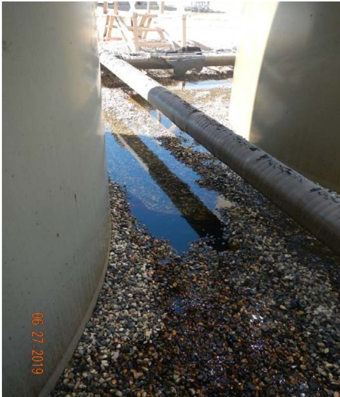
Photo#4: Pooling oil and staining in tank containment
