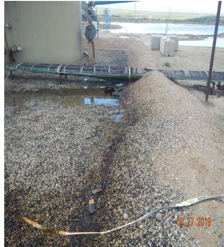
Photo#5: Pooling oil and staining in tank containment
