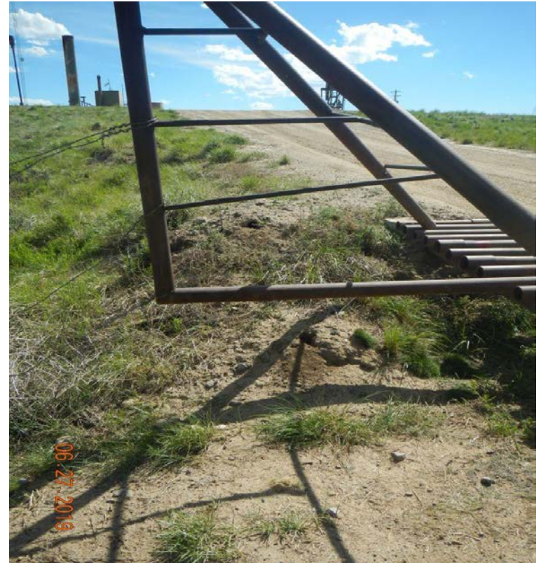
Photo#12: Lack of BMPs at Cattle guard entry.
