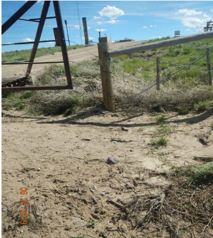
Photo#11: Lack of BMPs at Cattle guard entry.
