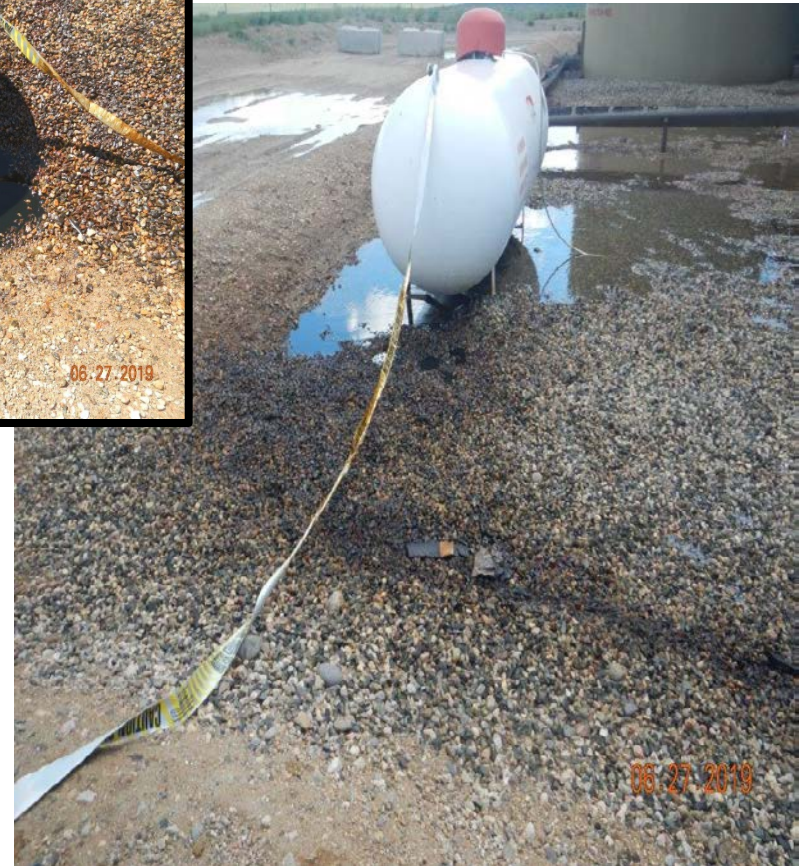
Photo#3: Pooling oil and staining in tank containment
