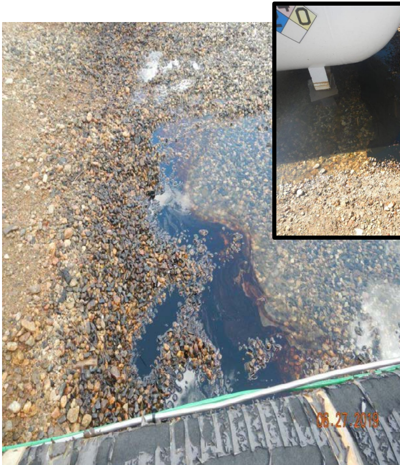
Photo#2: Pooling oil and staining in tank containment.
