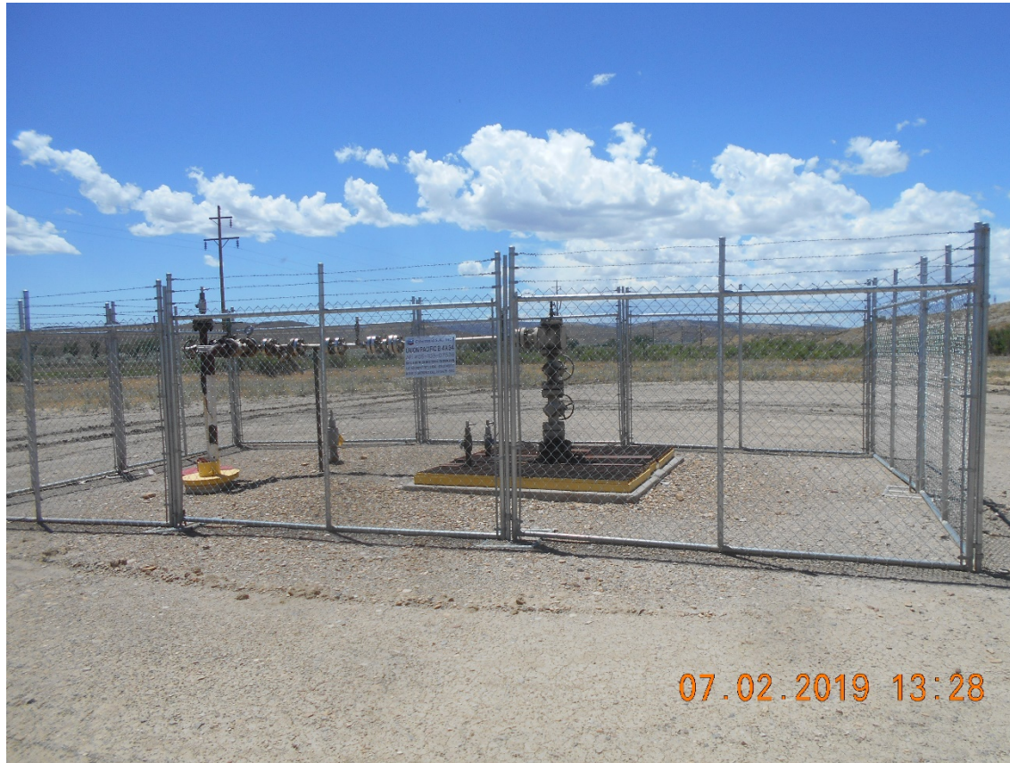
Injection Wellhead
