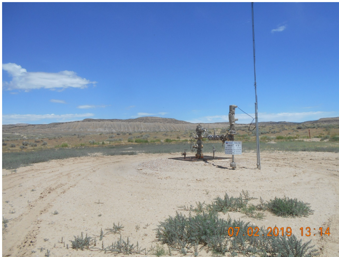
Injection Wellhead
