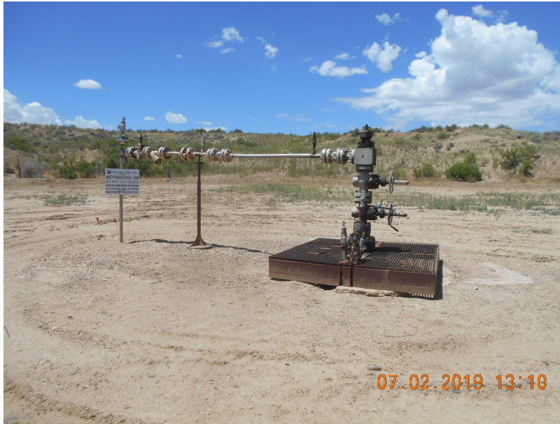
Injection Wellhead
