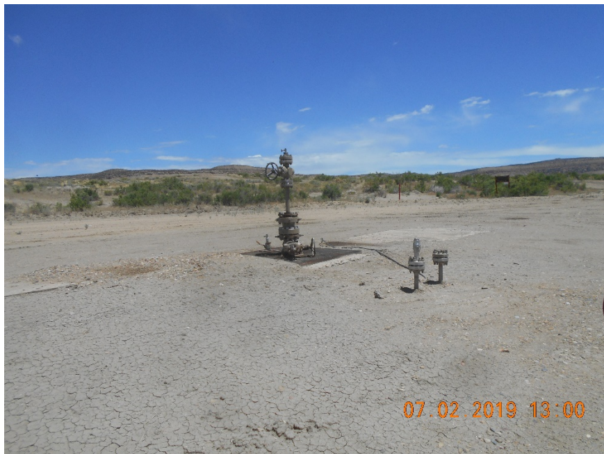
Injection Wellhead – Temporarily Abandoned
