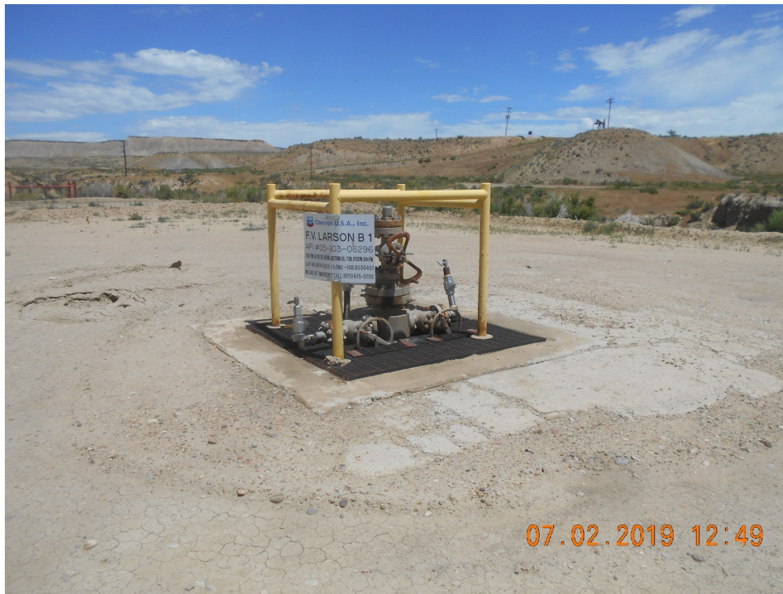
Injection Wellhead – Temporarily Abandoned
