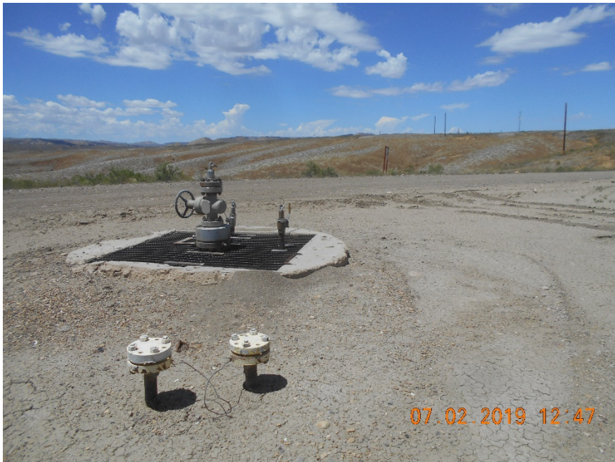
Injection Wellhead-Temporarily Abandoned
