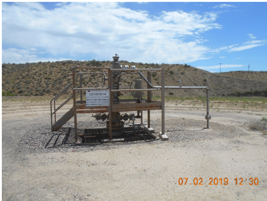
Injection wellhead
