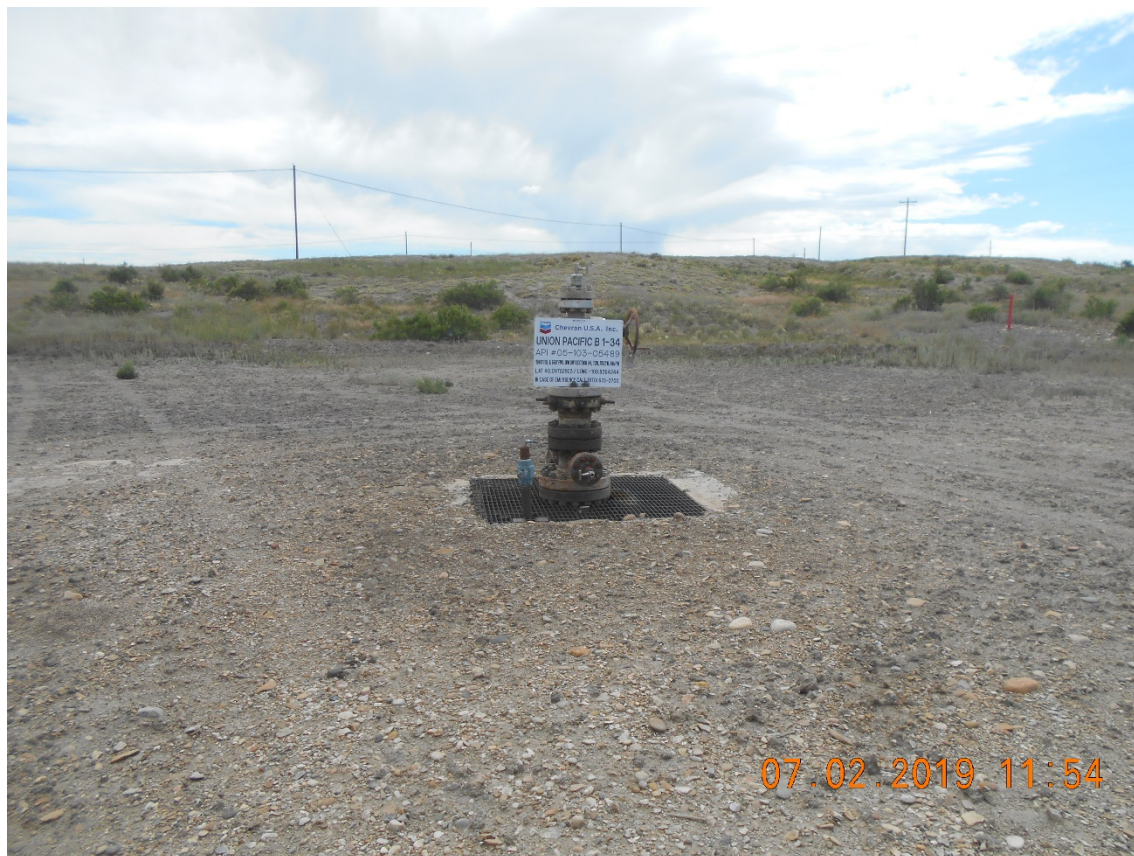
Injection wellhead – Temporarily Abandoned.
