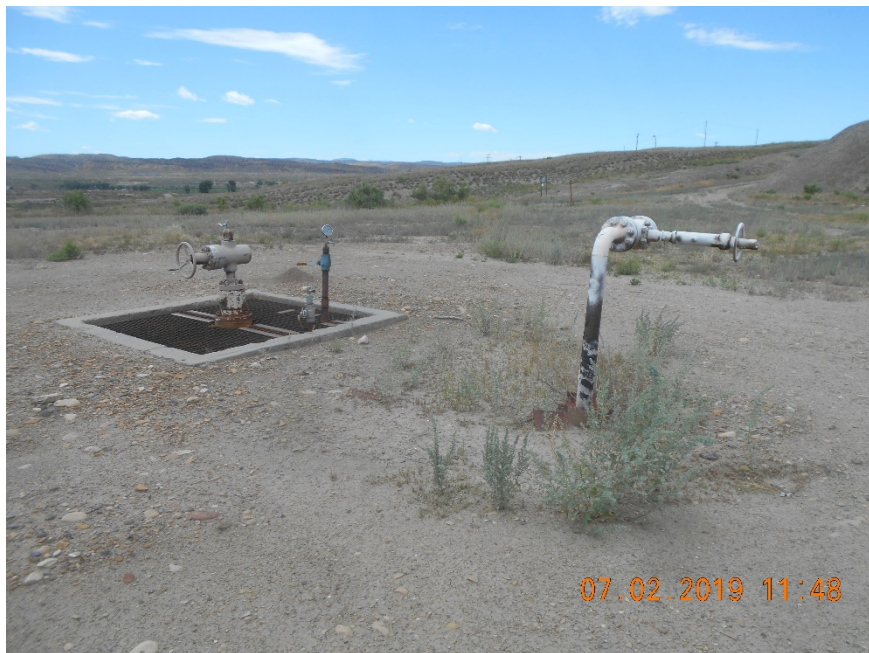
Injection wellhead – Temporarily Abandoned
