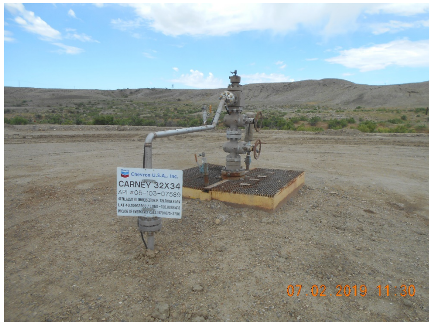
Injection wellhead
