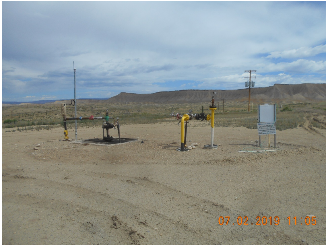
Injection wellhead converted to producer.
