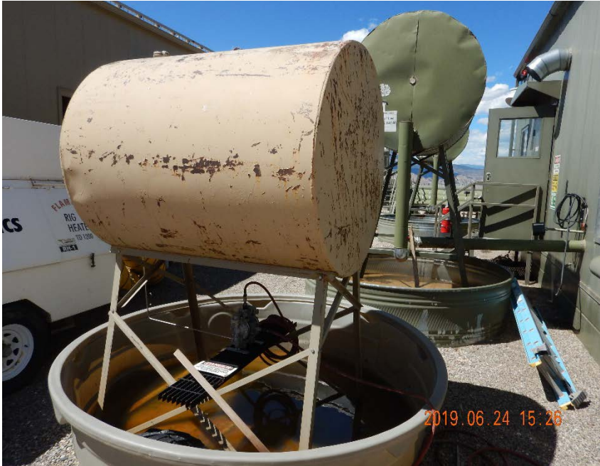
Photo #9 – Chemical storage tanks with secondary containment devices at compressor station (1).
