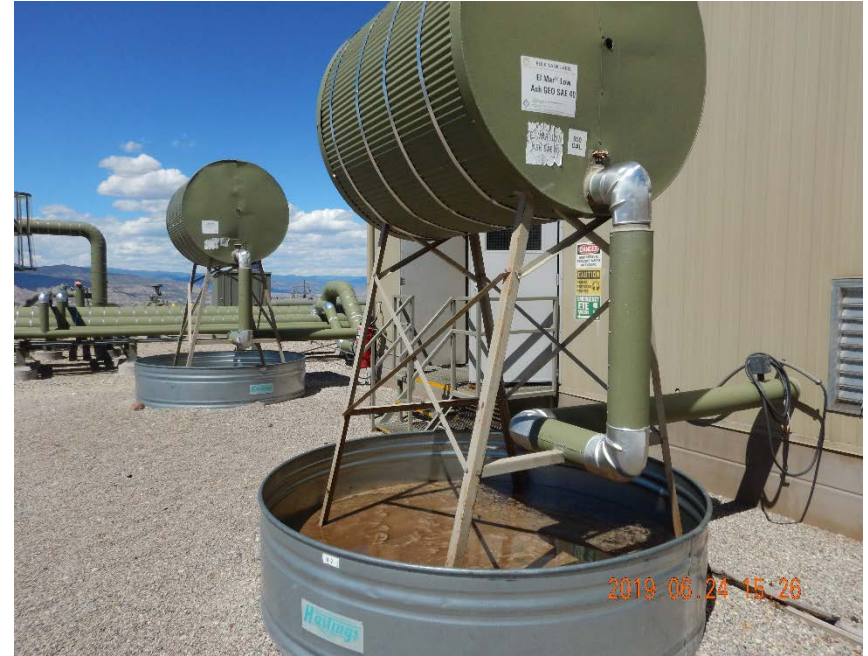
Photo #10 - Chemical storage tanks with secondary containment devices at compressor station (2).
