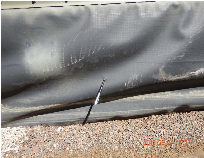
Photo #7 – Compromised section of tank battery liner on east side of battery.
