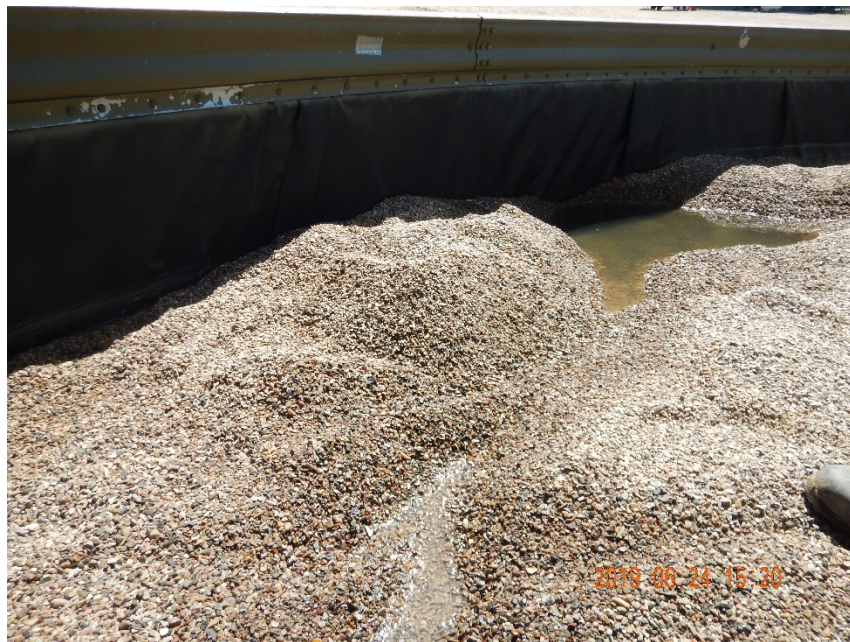
Photo #3 – Fluid remaining inside of tank battery berm on south side.
