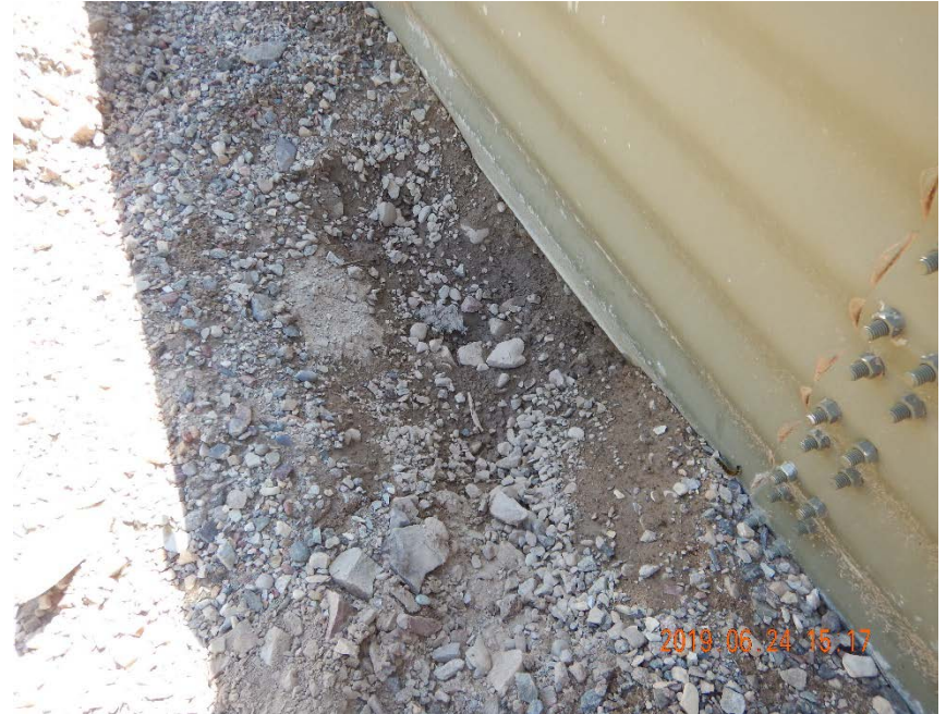
Photo #6 – Saturated area outside of tank battery containment berm on east side.
