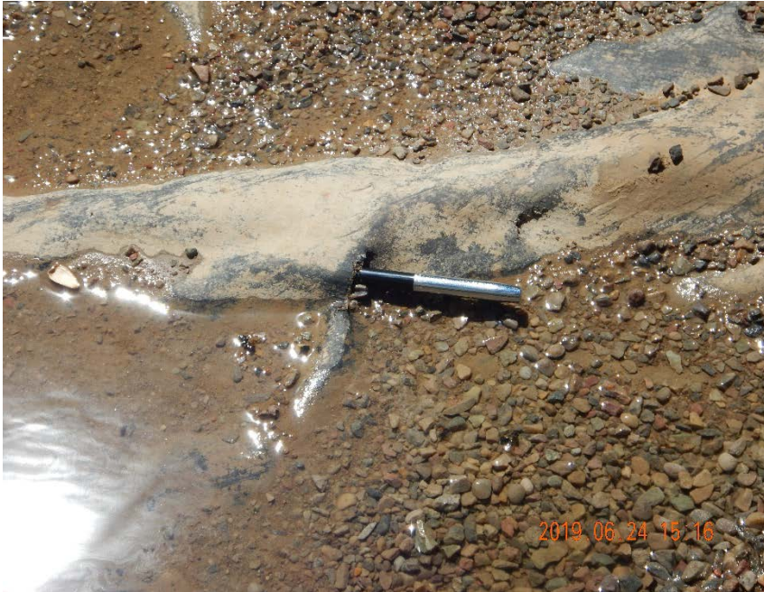
Photo #5 – Compromised sections of tank battery liner along base of containment area, east of tanks.
