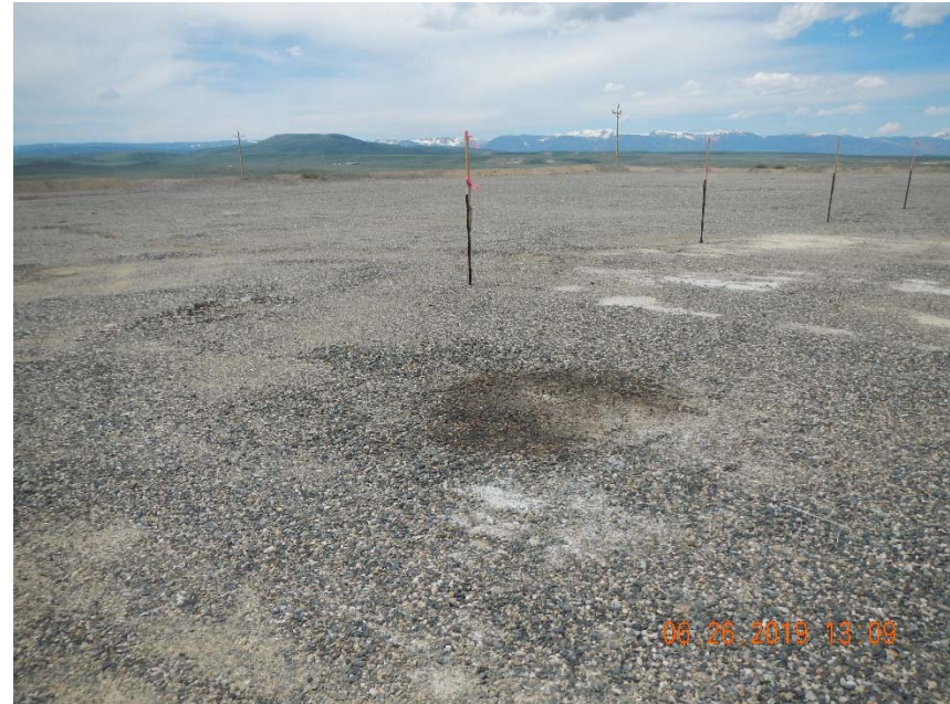
Photo 14. Frack sand spilled on location and an example of soil staining seen on entire location.
