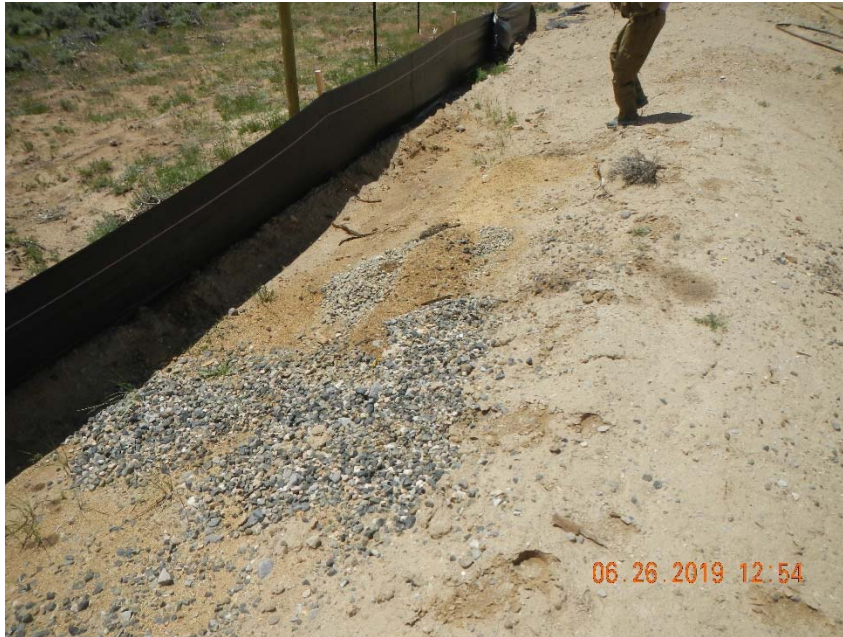
Photo 5. Drilling material pushed off edge of perimeter berm.
