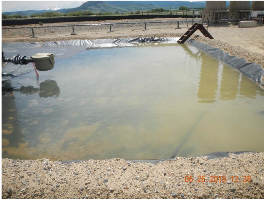
Photo 3. Stormwater in condensate tank berm.
