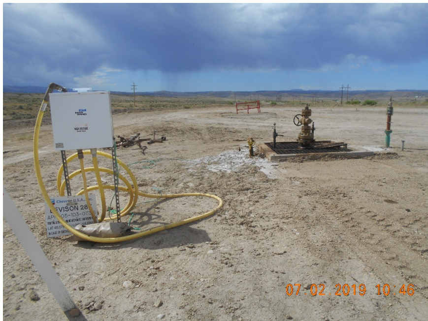
Injection wellhead-Temporarily abandoned. Production equipment (USP) on location and disconnected.
