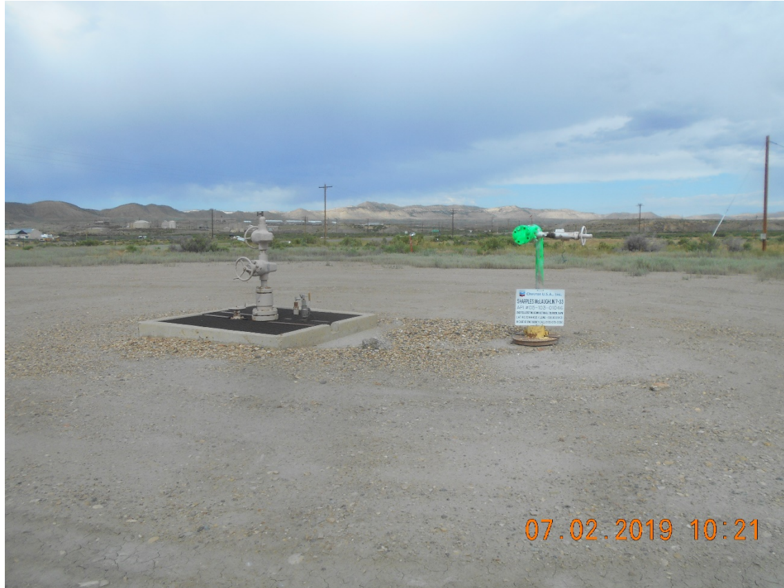
Injection Wellhead – Temporarily Abandoned
