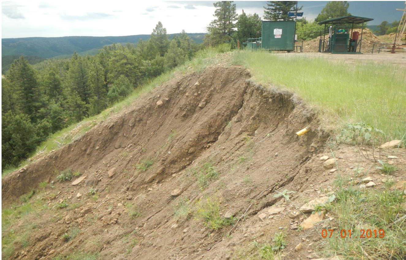
Photo 3. There is soil sloughing that occurred at the east side of the location.
