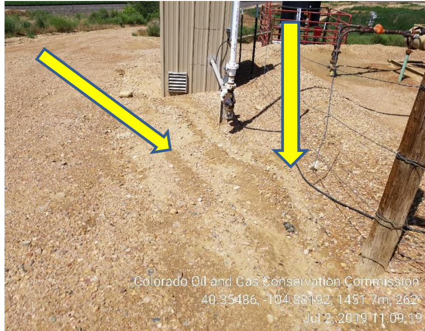
Photo 5: Erosion south of seperator
