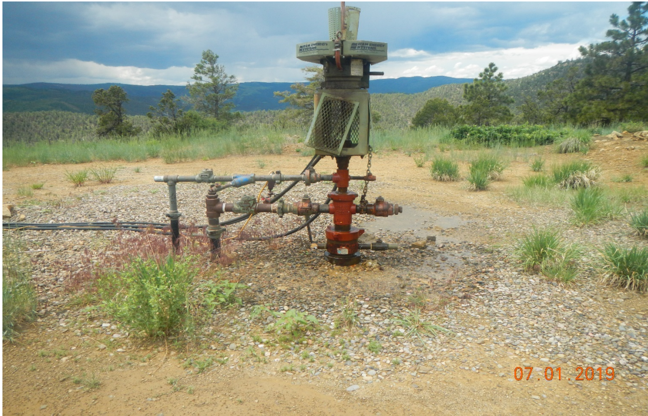
Photo 1. There is a dripping water leak from the wellhead.
