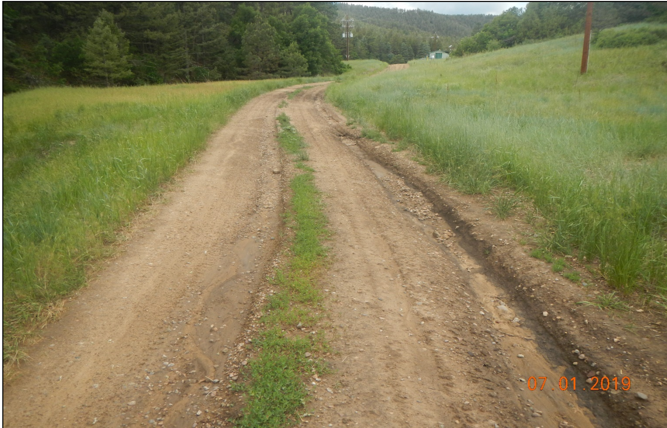
Photo 4. Vehicle ruts remain along the road which is a conveyance for stormwater erosion.
