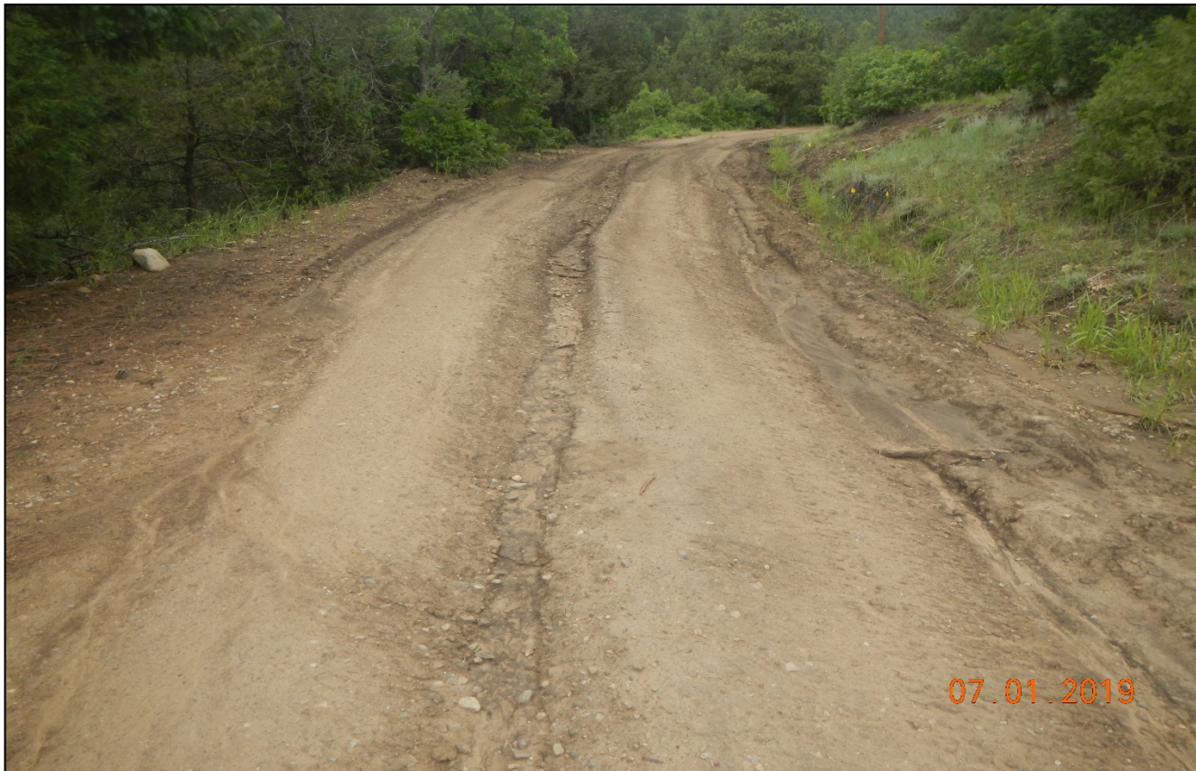
Photo 3. Vehicle ruts remain along the road which is a conveyance for stormwater erosion.
