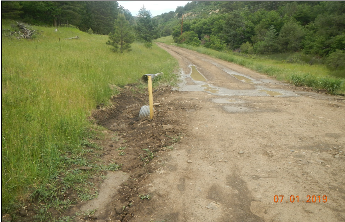
Photo 2. There were culverts cleaned out along the road. Scrap pieces of culvert remain near the culverts.
