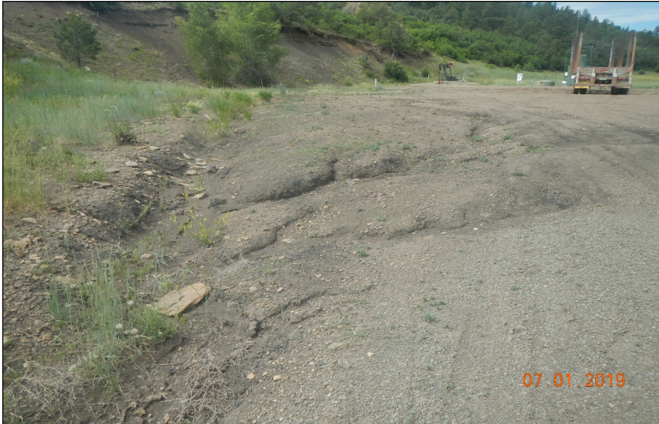
Photo 3. Facing southwest toward the location. There are erosion issues coming off the pad surface and is depositing sediment into the culvert along the access road.
