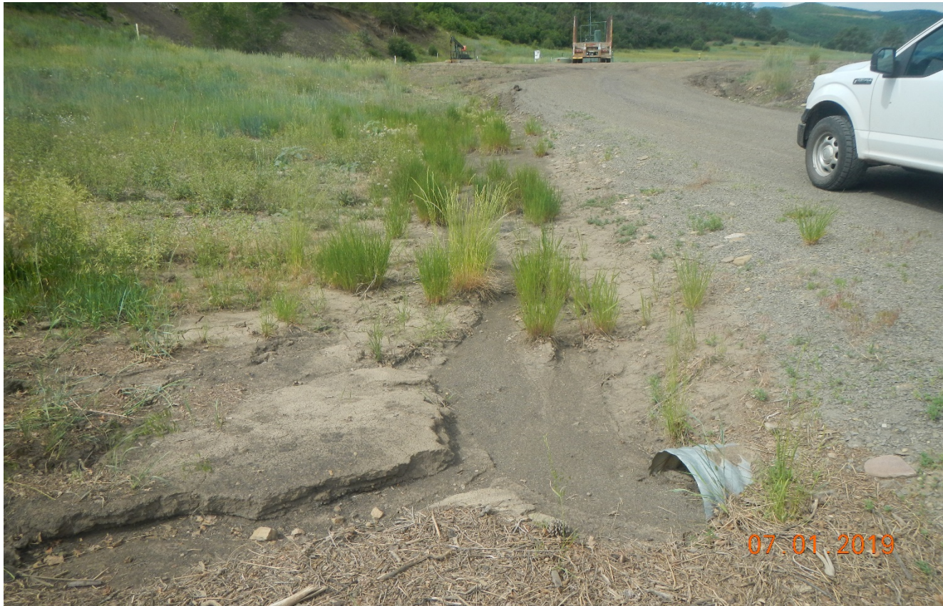
Photo 2. The culvert near the location is half full of sediment.
