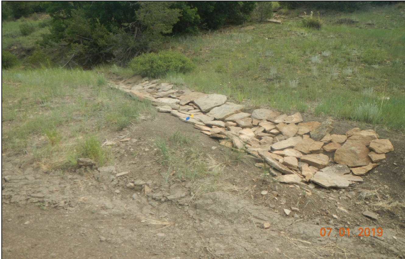
Photo 3. Rock rip/rap was placed in drainage channel.
