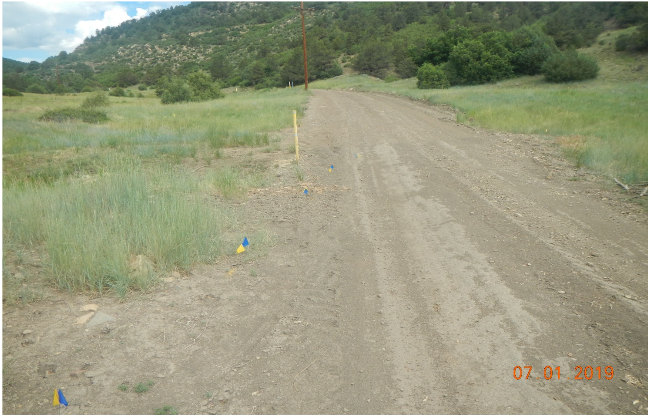
Photo 1. Facing northwest at mouth of the canyon.
