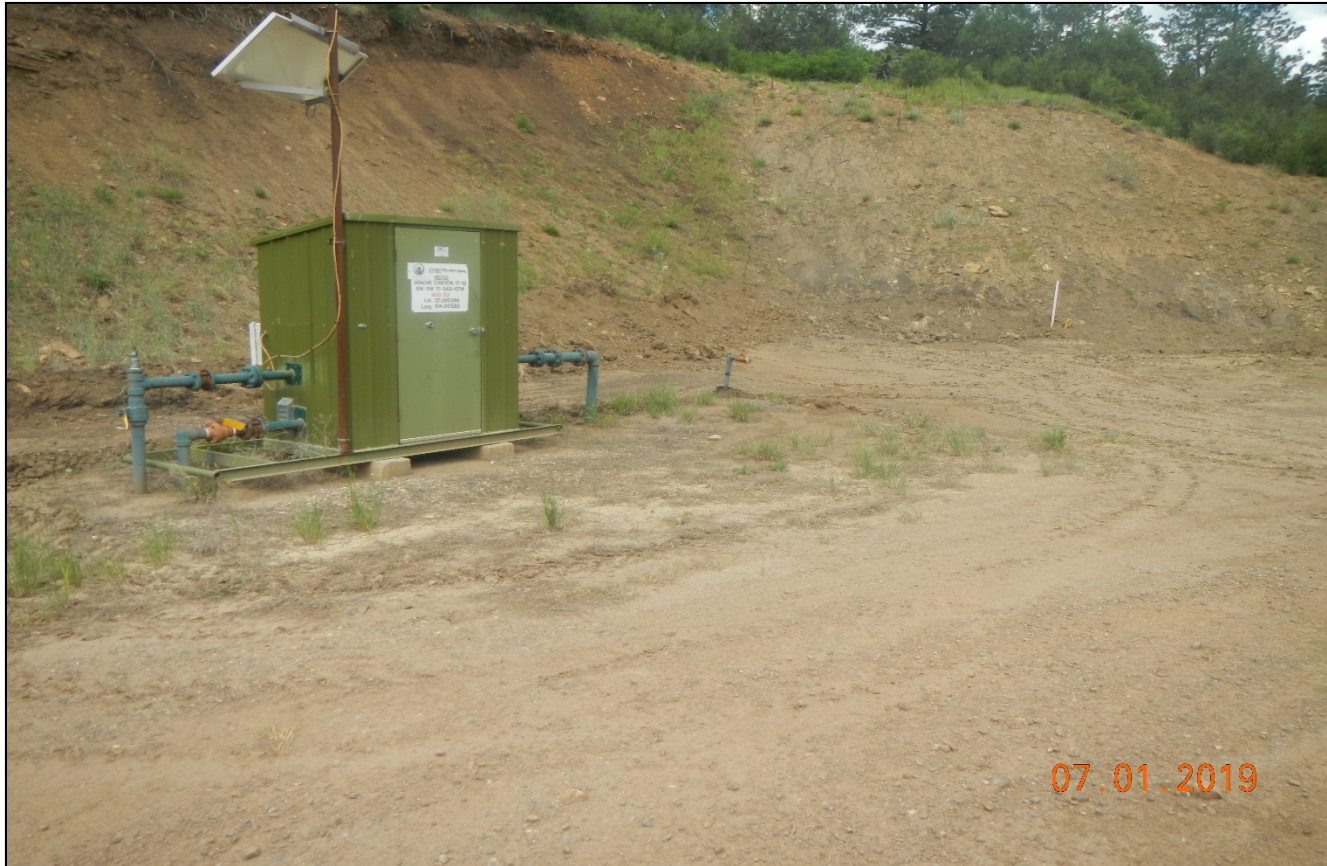
Photo 6. Facing toward the location. Sediment has been removed behind the equipment.
