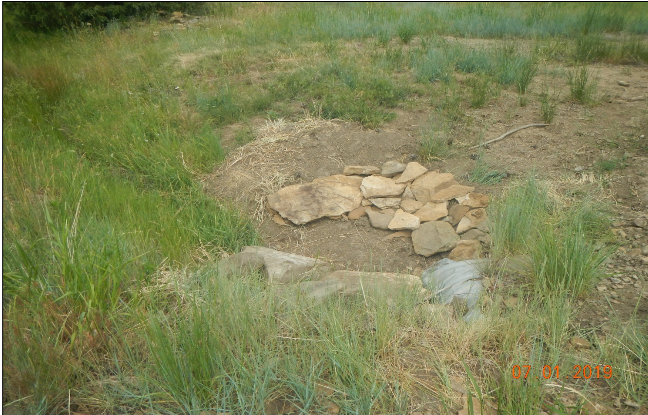
Photo 2. Culvert has been cleaned out since previous inspection.
