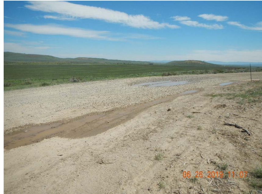
Photo 6. Gravel added to washout observed on 5/3/2019.
