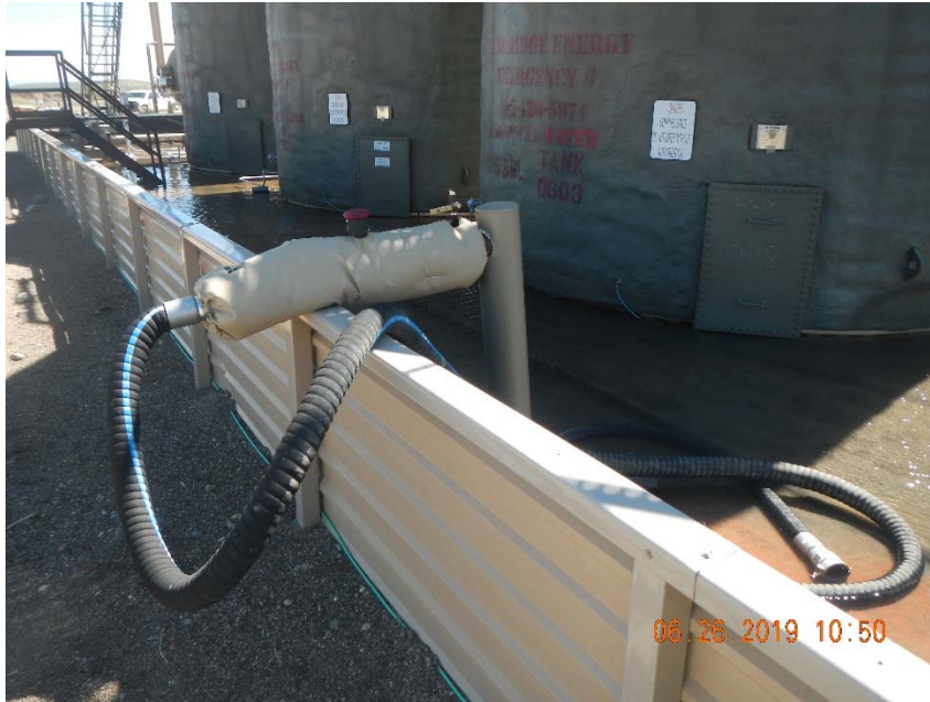
Photo 5. Stormwater in berm with loadout hose resting in water.
