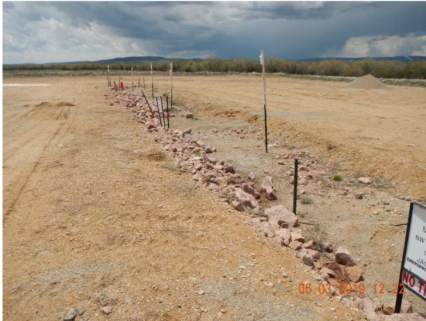
Photo 3. All wellheads buried in gravel.
