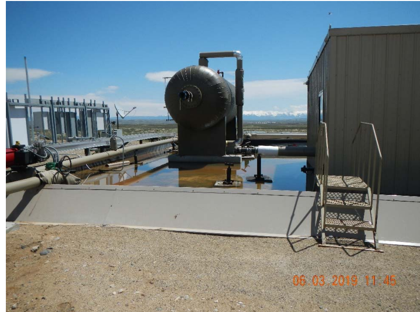
Photo 4. Unused triplex jet pump with secondary containment holding stormwater.
