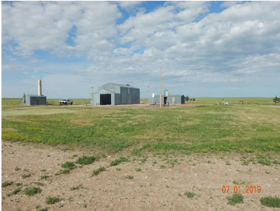
Photo 15: Photo taken from the north east end of the location, facing west. Photo shows equipment remaining on the location, and location has not been reclaimed.
