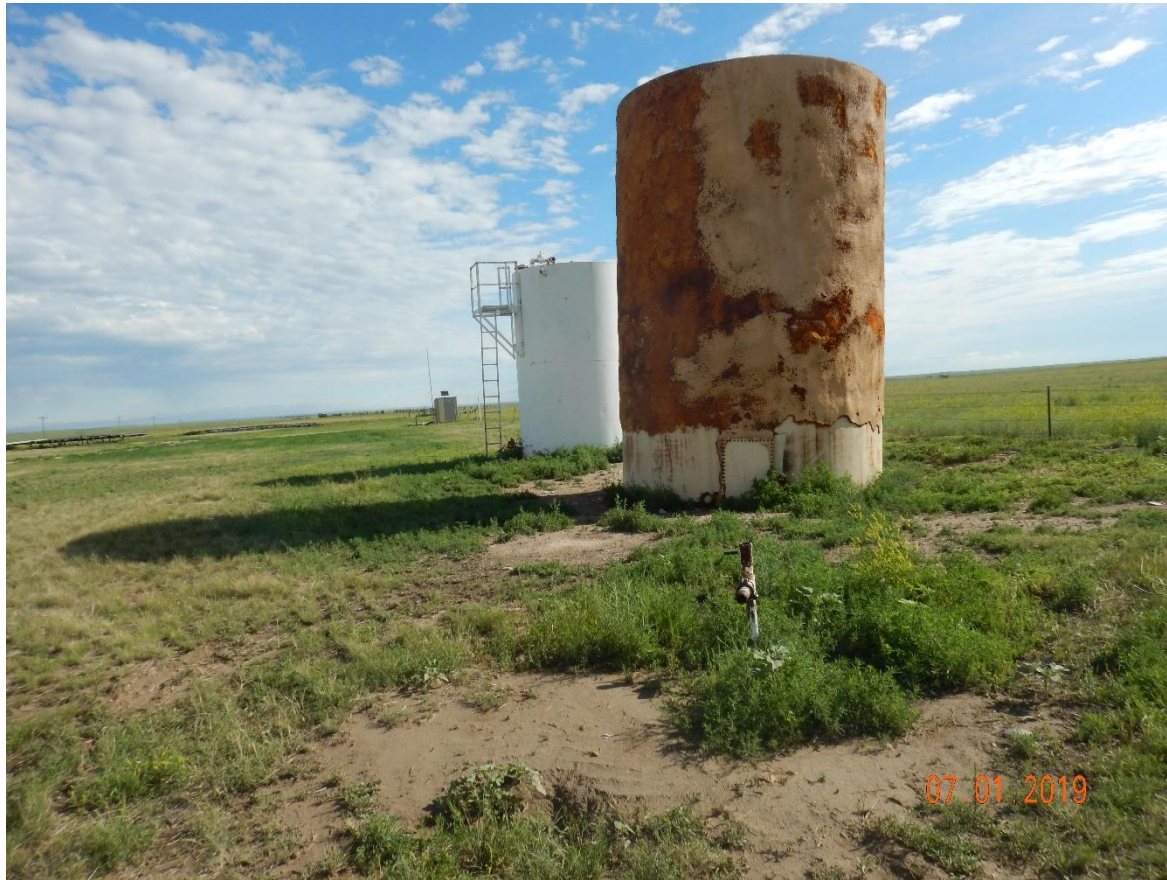
Photo 8: Photo taken from the southeast end of the location. Photo shows equipment has not been removed from the location, and location has not been reclaimed.
