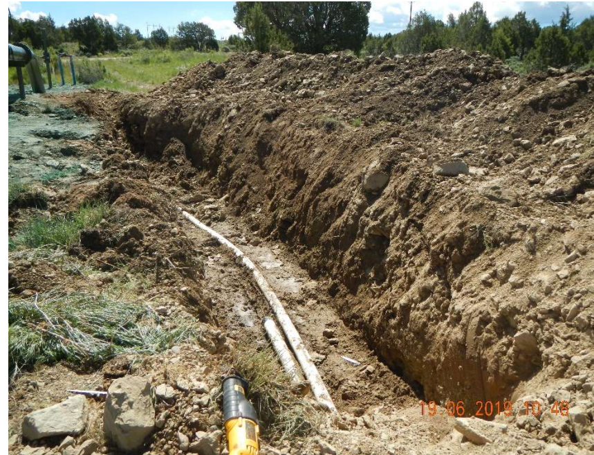
Photo #2 – View of the excavation and stockpiled soil looking north. The ruptured flowline can be seen in the bottom of the excavation.
