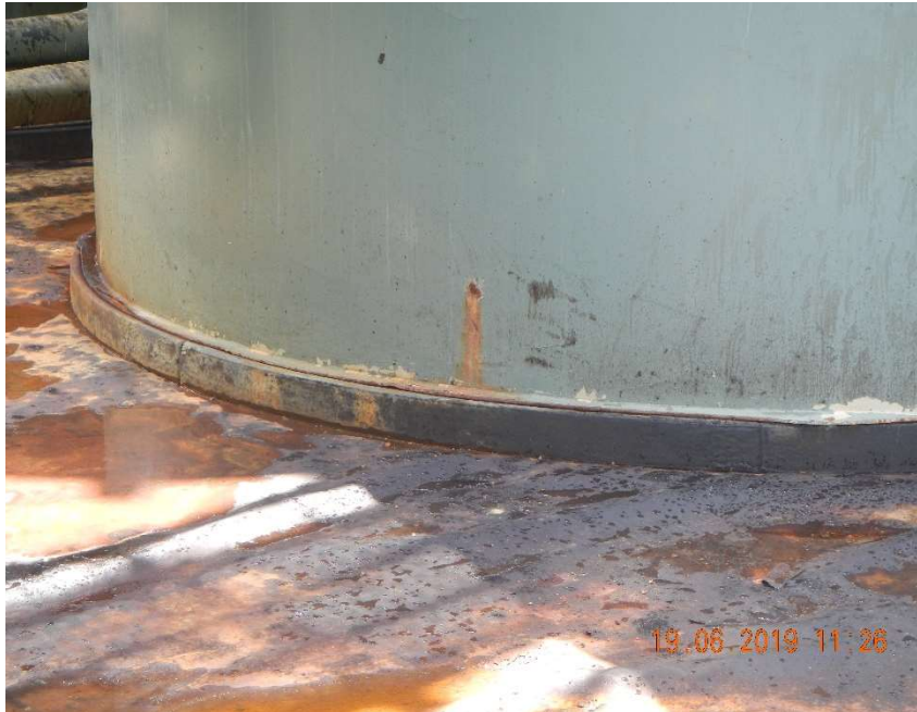
Photo #5 – View of the pen sized hole in one of the 500 BBL produced water tank.
