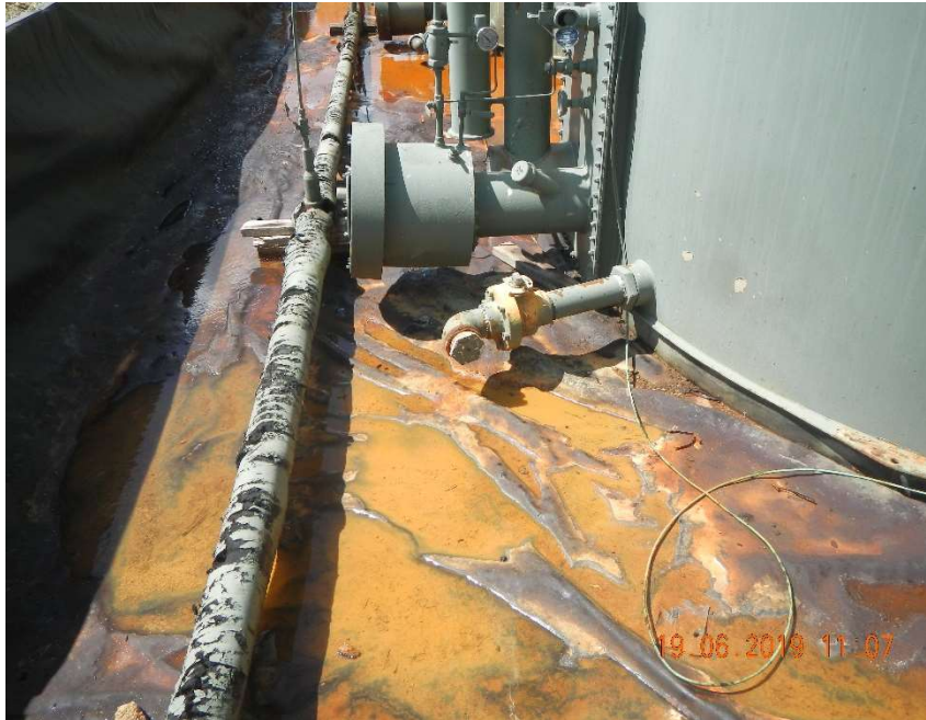
Photo #3 – View of the dripping plug and the impacted storm water.
