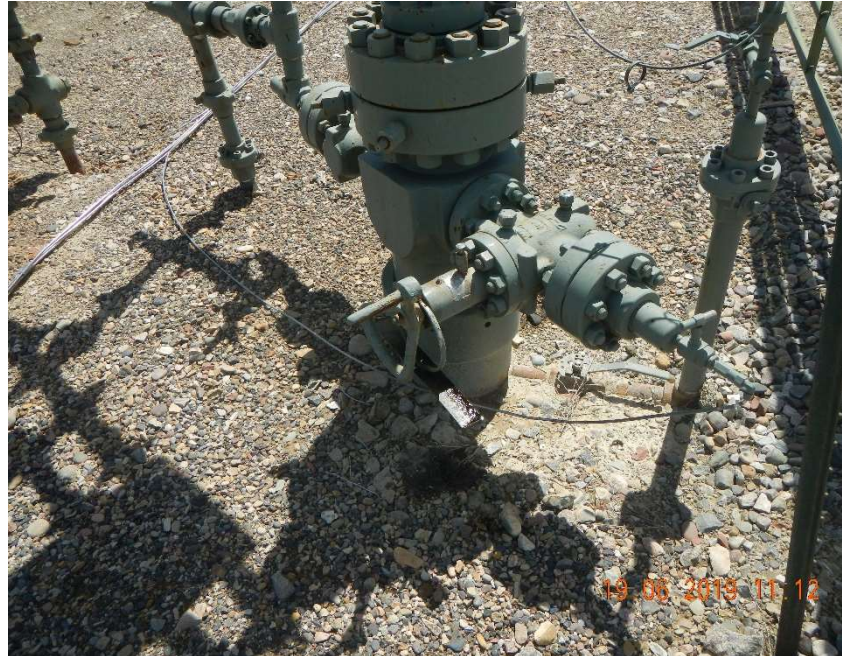
Photo #7 – View of the leaking well head.
