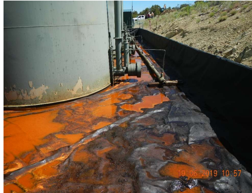
Photo #4 – View of the stained pit liner and impacted storm water.
