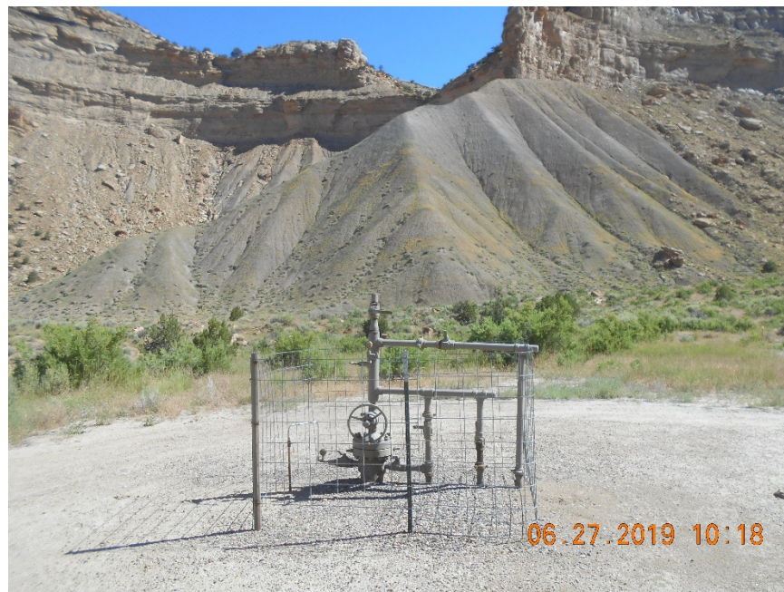
Wellhead with fence
