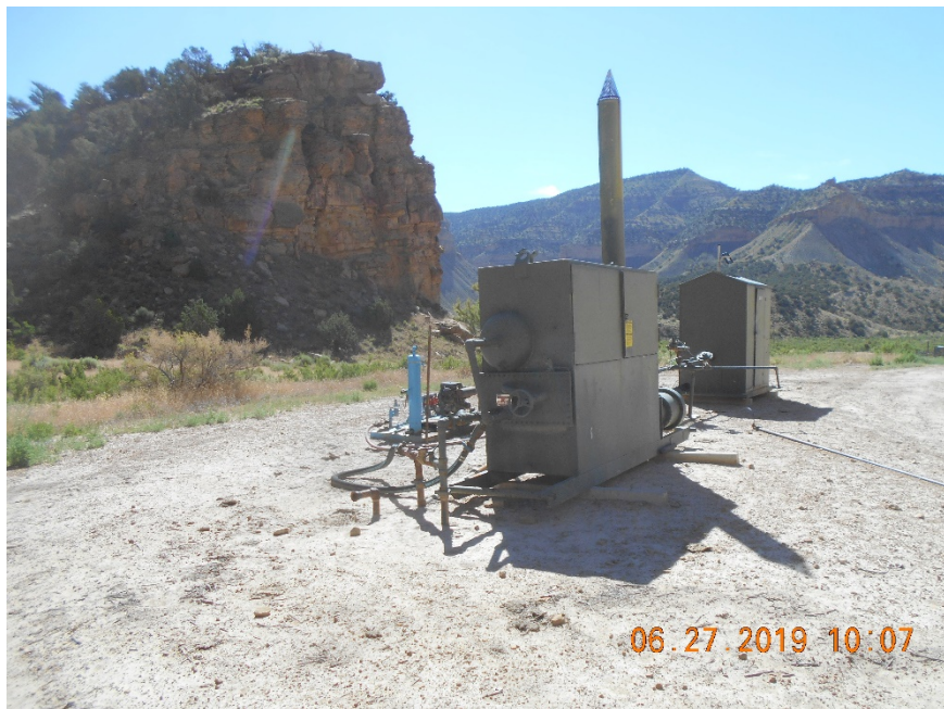
Separator and Meter housing.
