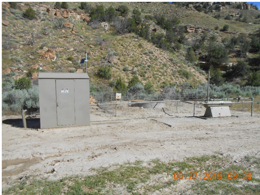
Meter housing , Separator and Blowdown tank with fence.
