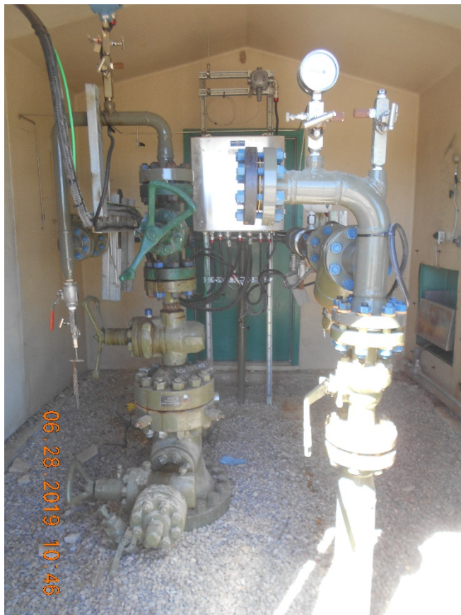
Injection wellhead inside housing
