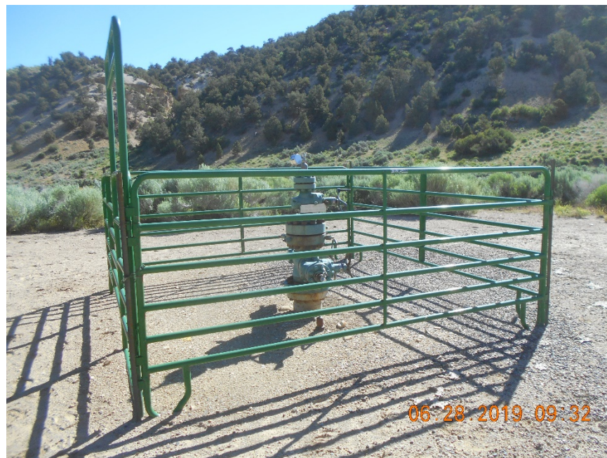
Injection Wellhead Temporarily Abandoned
