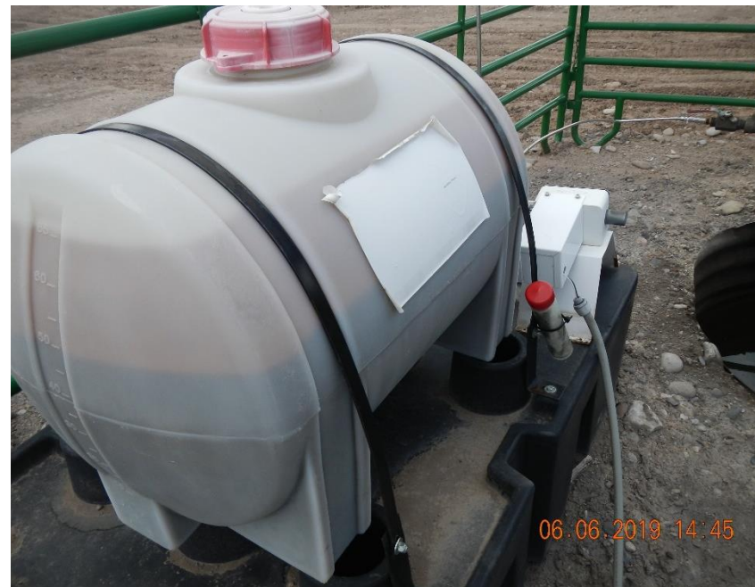
Illegible label on chemical injection system for #3 well head.
