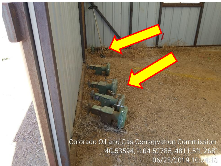
Photo 5 – Unused Pneumatic Injection Pumps in East Engine house, along South wall
