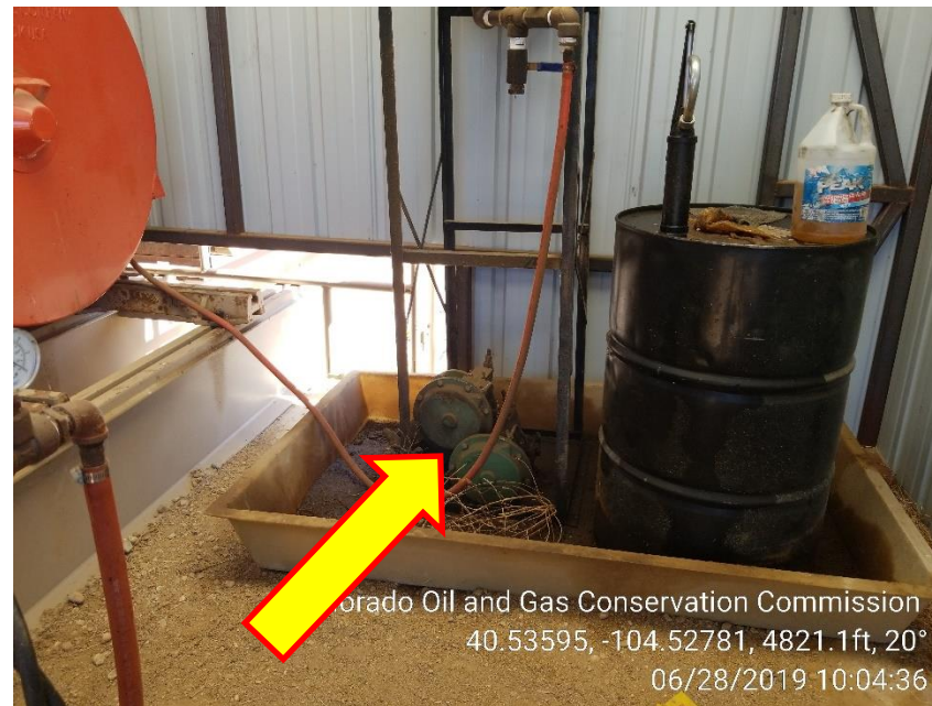
Photo 6 – Unused Pneumatic Injection Pumps in East Engine house, along North wall
