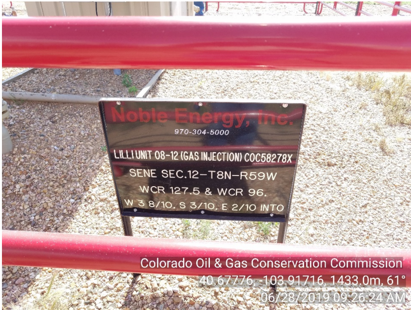
Photo #1 Lilli Unit 8-12 (05-123-13865) UIC - Injection Wellsite UIC Annual Inspection Shut-In | SI Not Injecting
