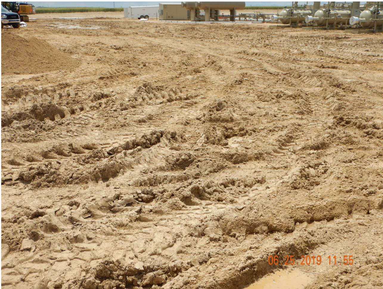
Photo 6. Photo taken from the southern pad, facing East. See comments under Photo 5. Photo also illustrates rutting throughout the location which the Operator is tracking off location because there are no vehicle tracking device BMPs at either of the entrances. The vehicle tracking device has only been installed at the intersection of CR 15.
