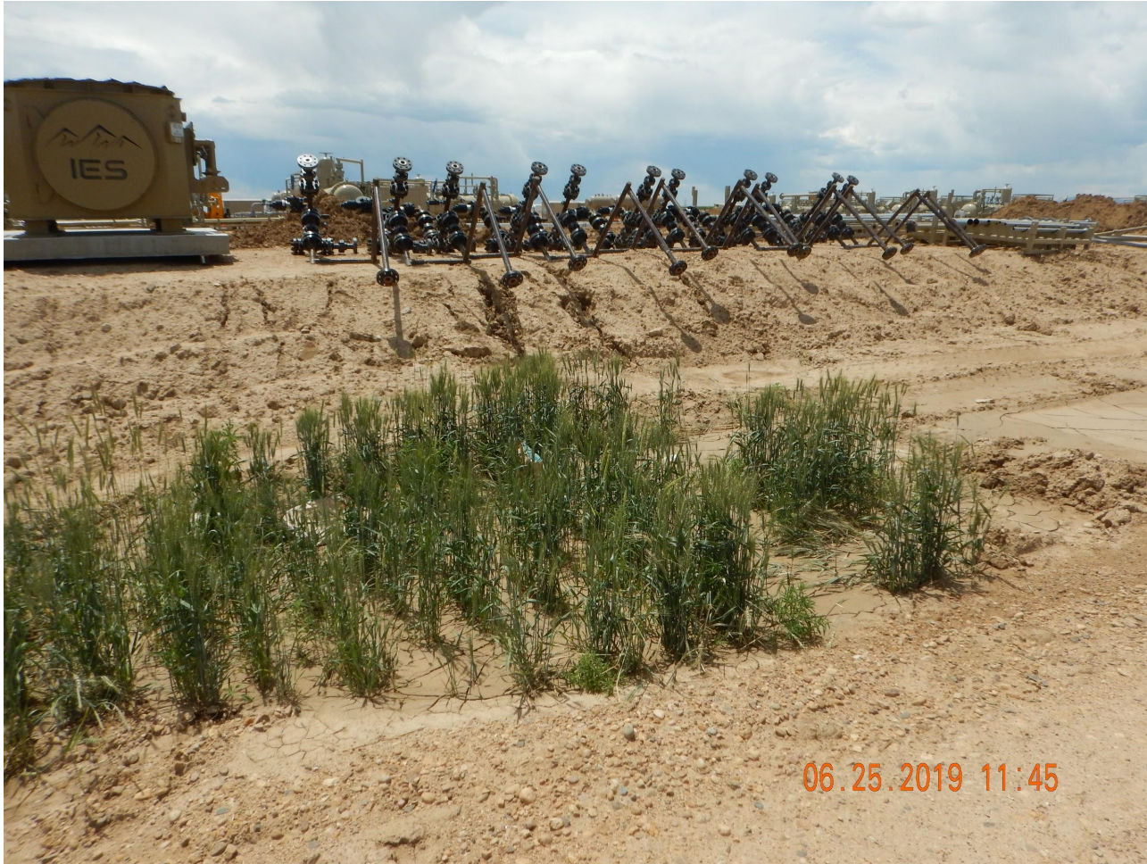
Photo 5. Photo taken of the fill slope of the southern pad, facing South. Photo illustrates the Operator has failed to maintain the location so as to reasonably minimize erosion, and site degradation per Rules 1002.e. and 1002.f.
