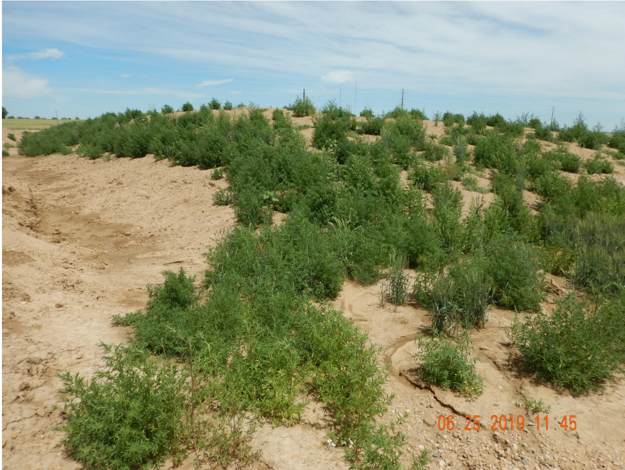
Photo 1. Photo taken of the northern topsoil stockpile, facing North. Photo illustrates the Operator has failed to protect the topsoil from erosion and weed establishment. Weeds were approximately 3' tall and erosion was observed throughout the stockpile.
