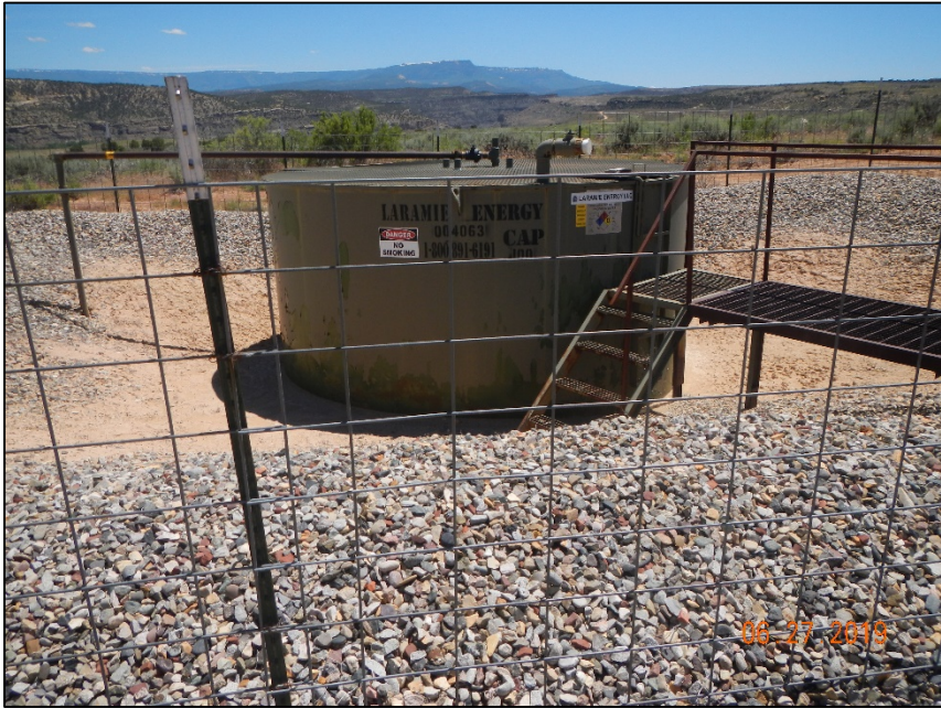
Photo # 3 Photo of Tank Battery
