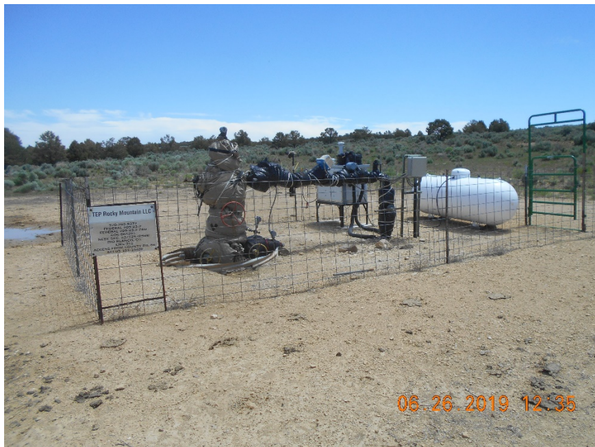
Injection wellhead & line heater
