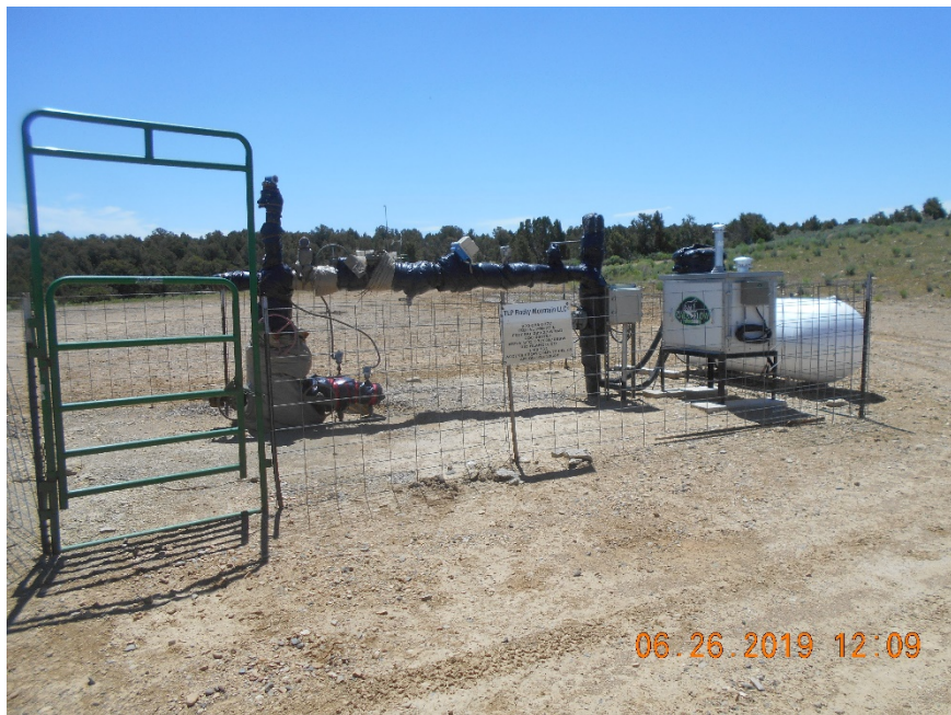
Injection wellhead & line heater
