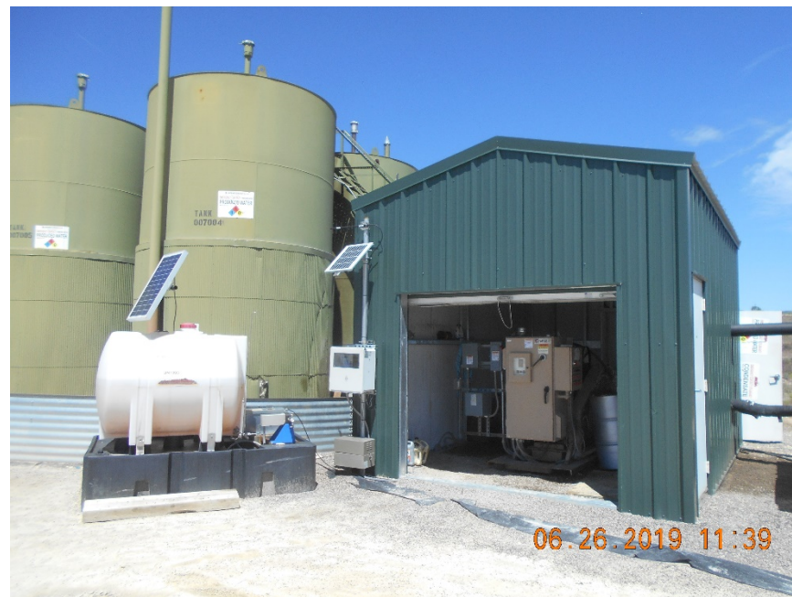
Pump Housing. Chemical injector with secondary containment.
