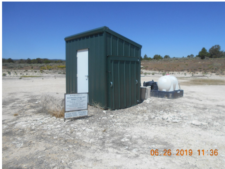
Injection wellhead inside housing. Chemical injector with secondary containment.
