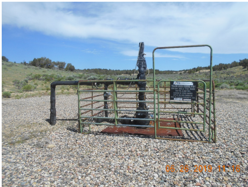
Injection wellhead
