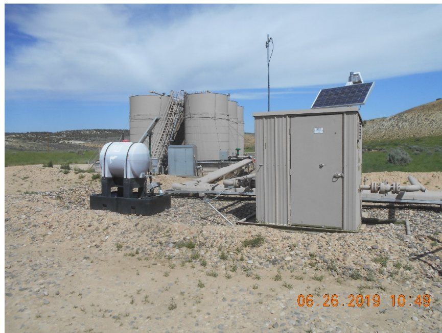
Meter Housing. Chemical containers with secondary containment.
